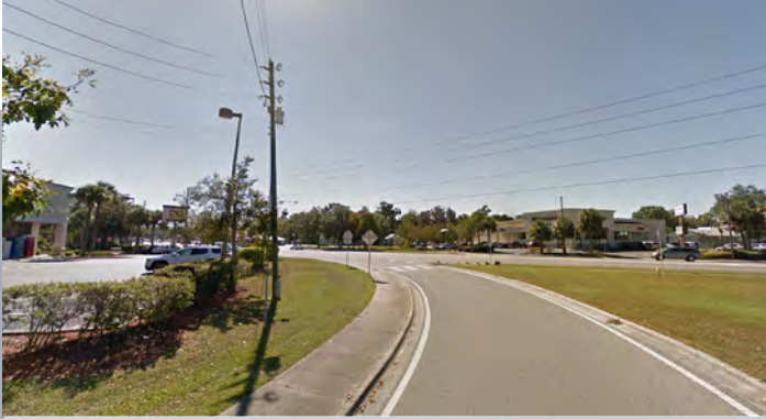
Intersection of US 19 / US 98 and SR-44 Existing
