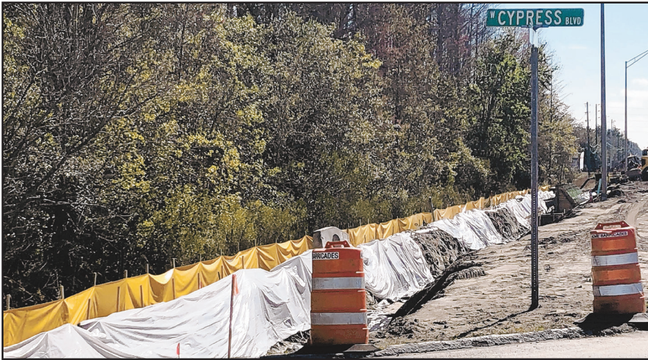
The construction of the 10-foot-wide multipurpose path is getting close to the Sugarmill Woods Cypress Village entrance. Portions of the path will include conduit to protect electric lines to control stop lights and other utilities. The creation of this path designed for pedestrians and cyclists will cost $2.8 million. (Gazette staff photo)
