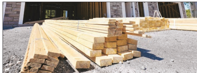
Lumber is piled at a housing construction site in Middleton, Mass.
