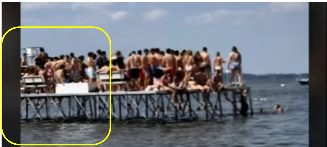
1) 1 Second before collapse all vertical support legs are currently vertical.
