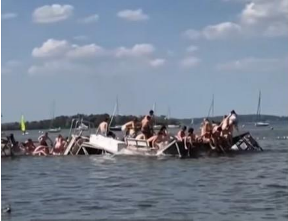
7) 2 Seconds in, pier support legs have finished failing in a cascade.
