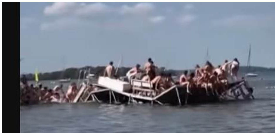
6) Extended failure continues across pier support legs and horizontal edging.
