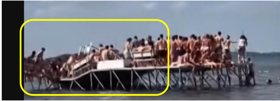
4) Continued cascade of support legs and deck edging failing northward.
