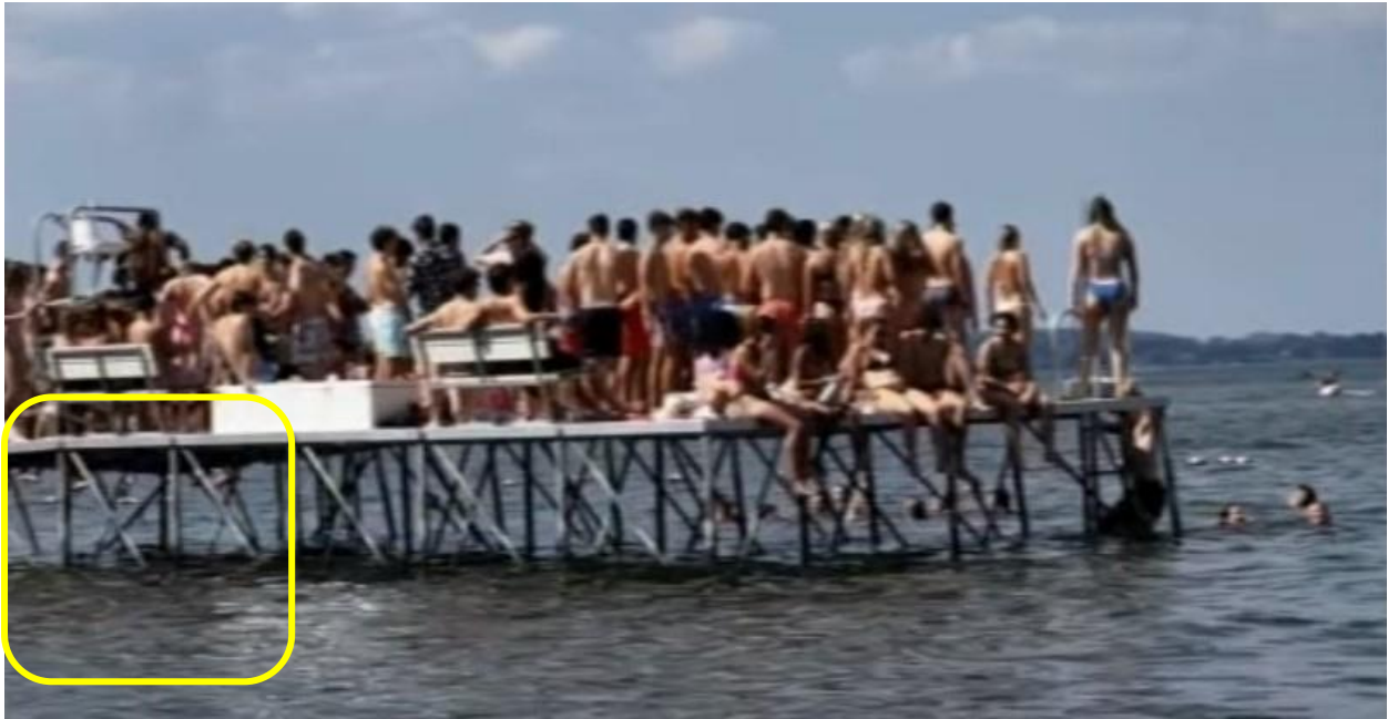
2) 0 Second. Failure begins. Notice bulge on the decking at the far left of this image, at the underside of the pier deck; the leg beneath that bulge appears to be buckling northward.
