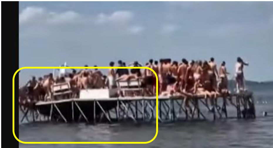
3) Less than .5 seconds later, multiple support legs have buckled in numerous directions and the horizontal edge of the pier decking is buckling across numerous sections. Occupants have begun falling into the water.
