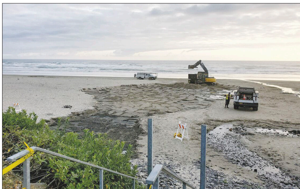
City crews were quick to secure and clean up the area last summer when a wastewater pump station failed spilling an estimated 26,000 gallons of sewage onto the beach.
