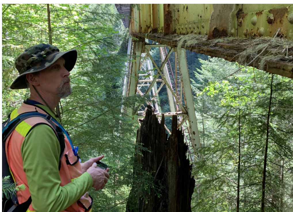
An engineer working where the rail line passes through the Tillamook State Forest. Photos provided by Jon-Paul Bowles
