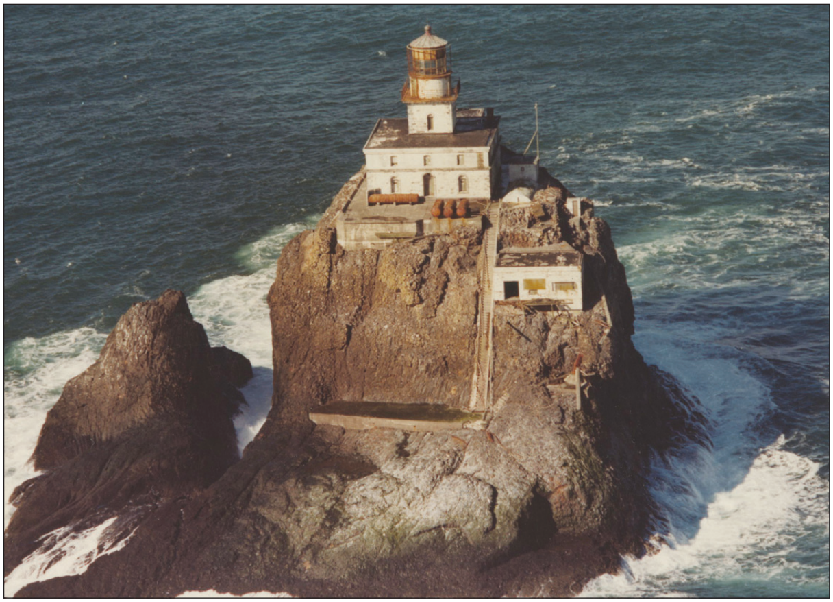
Tillamook Rock Lighthouse. Courtesy photo
