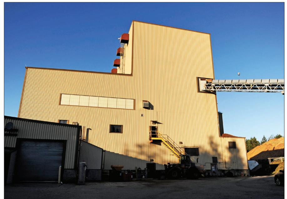
Biomass power plant DG Whitefield faces an uncertain future after proposed subsidies failed to materialize. (Photo by Paul Hayes)
