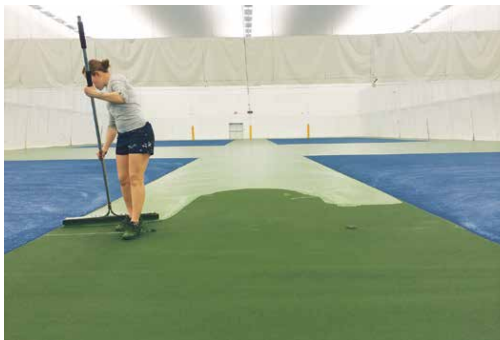
Nicquelle uses a giant squeegee to paint the surface of one of her tennis court projects.
