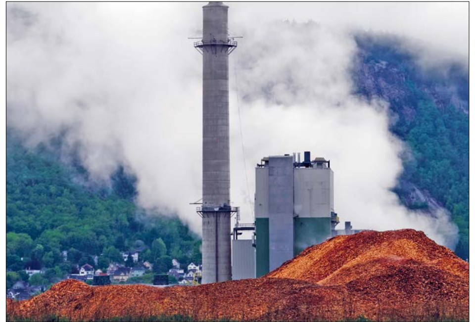
The biomass power plant in Berlin, N.H.
