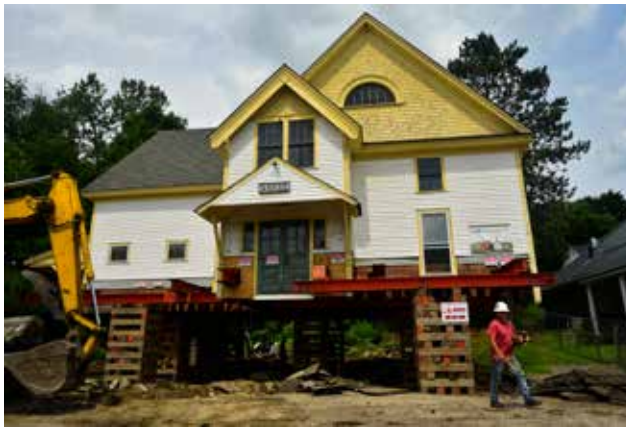
The Littleton Community Center, whose annex is pictured here raised in July so foundation work can proceed, is seeking a $500,000 Community Development Block Grant to advance major renovations. (Photo by Robert Blechl)
