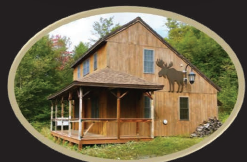
#4640292 – No roughing it! Modern kitchen, 3BR, full bath, dedicated generator, gas or wood heat, on 67A. $139,900. Contact Lyell.
