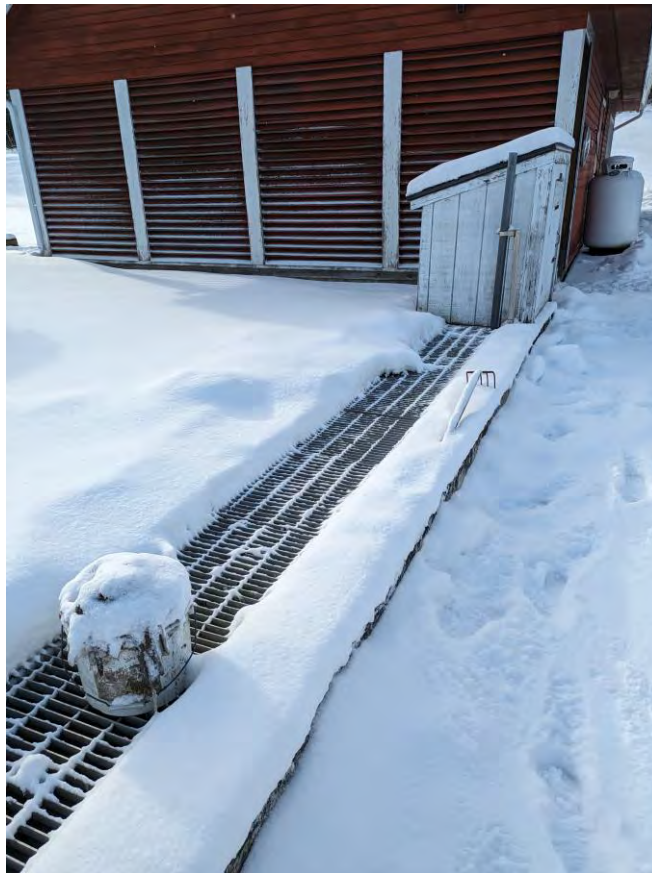
Figure 2-7: Headworks Channel & Influent Sampler
