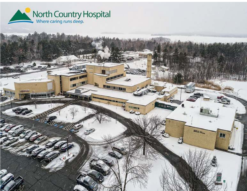
An aerial view of North Country Hospital in Newport City on its Prouty Drive campus.
