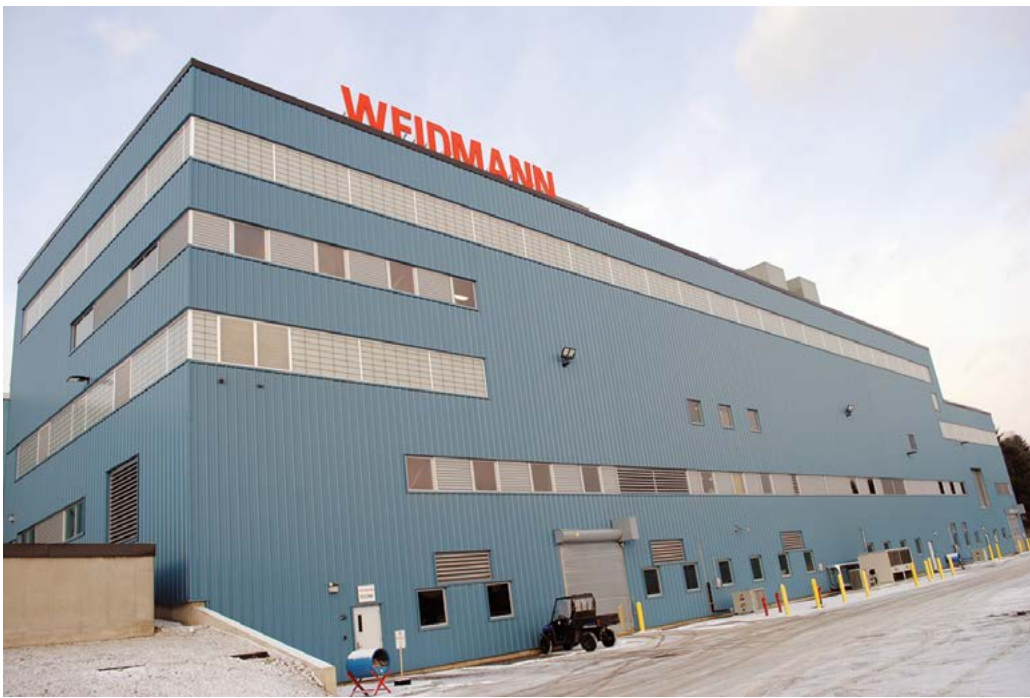
The Weidmann plant located on Route 5 in St. Johnsbury. (Photo by Todd Wellington)
