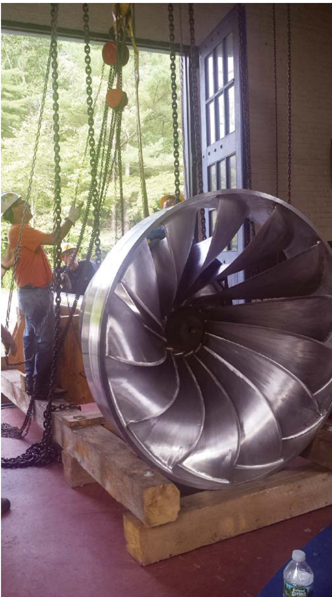
In this photo from August 2016, a crew from Fairbanks Mill works to install a new turbine runner at the Green Mountain Power Hydro Station. (Courtesy Photo)
