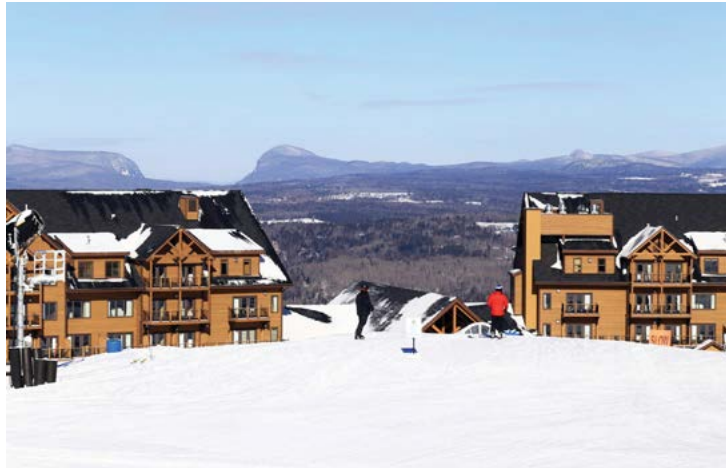
The new Burke Mountain Hotel & Conference Center in East Burke, Vermont.
