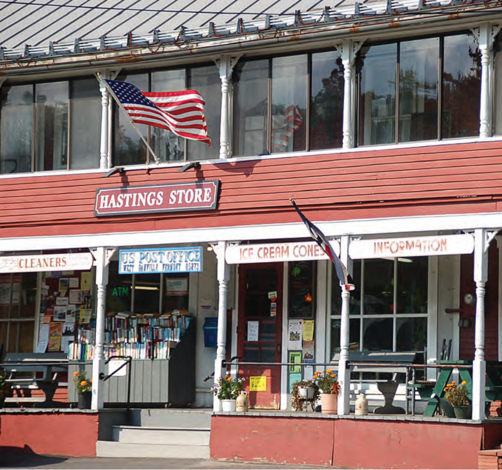
Hastings Store has been a fixture at the junction of routes 2 and 15 in West Danville for the last 105 years.
