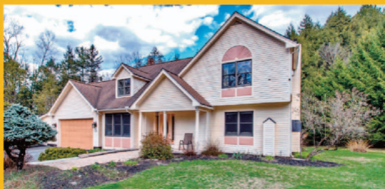
St Johnsbury: Thoughtful layout w/ exquisite details inside this 2,495 sq ft home on landscaped lot. Rachel. #5080582
