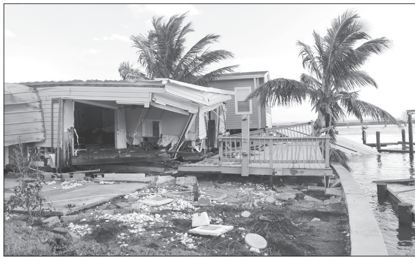
A home at Harbor Lights Club mobile home park in Pinellas County in the aftermath of Hurricane Helene on Friday, Sept. 27, 2024.
