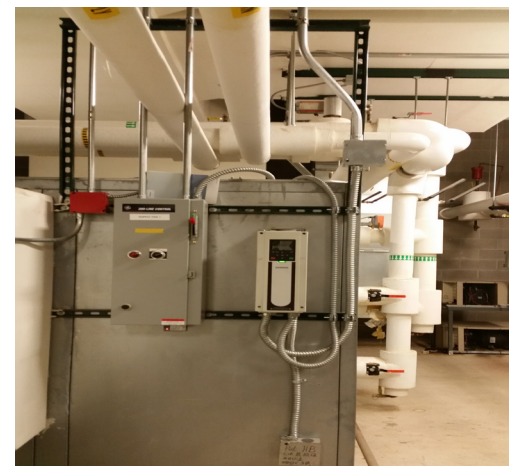
2017 digital controlled VFD air handler
