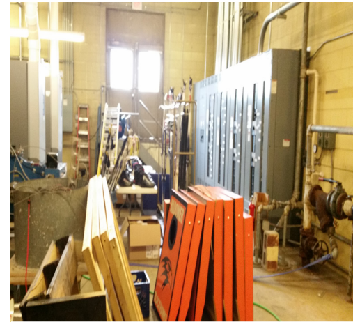
Improper mechanical room storage
