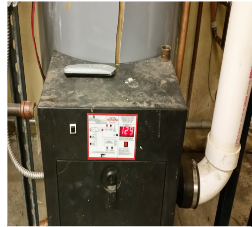
Domestic water heater temp control
