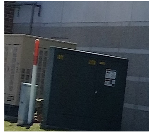
Unsecured transformer & generator
