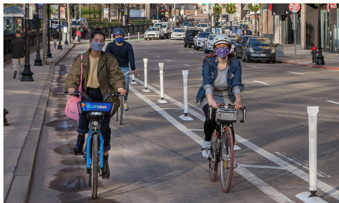
Example of a one-way separated bike lane in Boston, MA Source: Boston Cyclists Union
