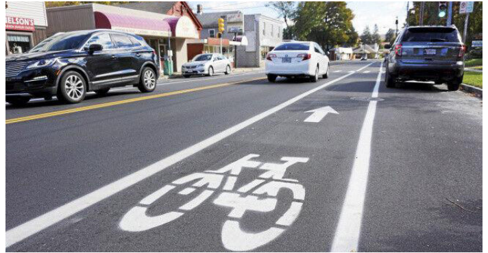
Bike lanes and Sharrows were added on Elm Street in 2015. Source: The Berkshire Eagle
