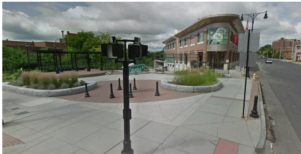
The Joseph Scelsi Intermodal Transportation Center in downtown Pittsfield. Source: Google Earth Streetview
