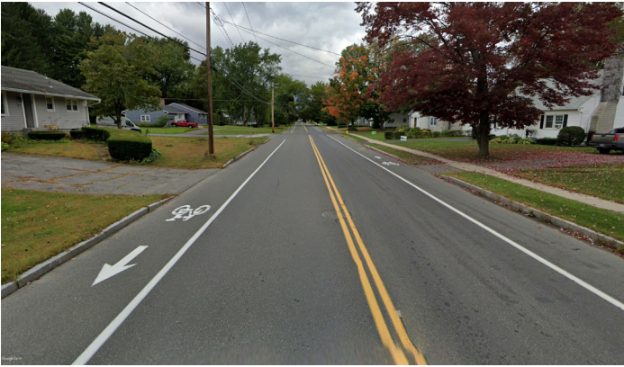
Elm Street: Example of LTS 2 Source: Google Earth Streetview
