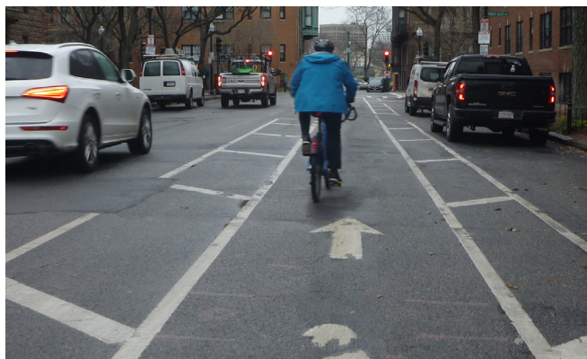
Example of a buffered bike lane adjacent to on-street parking in Boston, MA Source: City of Boston, MA
