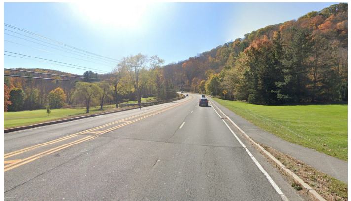
South Street: Example of LTS 4 Source: Google Earth Streetview
