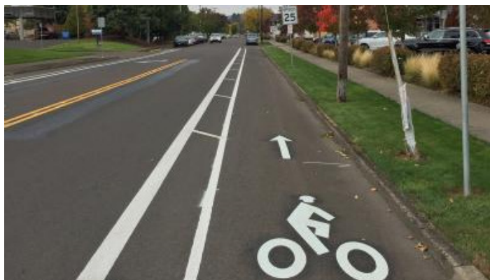
Example of a buffered bike lane in Corvallis, OR. Source: City of Corvallis, OR
