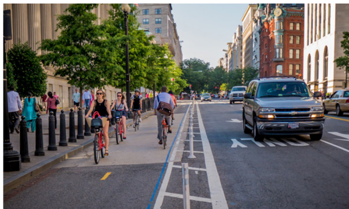
Example of a Two-Way Separated Bike Lane in Washington DC Source: People for Bikes
