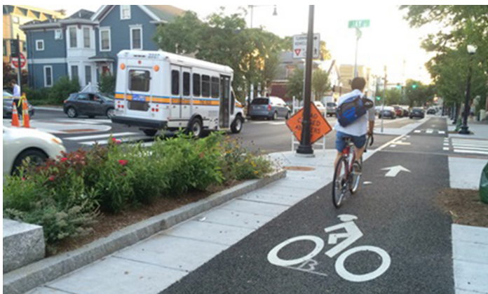
Example of a one-way separated bike lane in Cambridge, MA Source: City of Cambridge, MA
