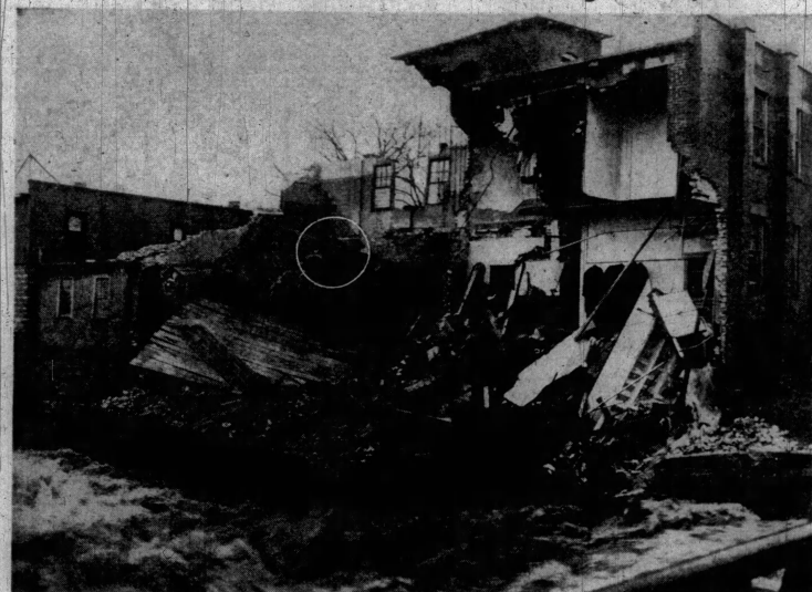
Photo shows rear of Petri Cleaning and Dyeing firm building at River and Eagle streets which collapsed yesterday afternoon and (circled), clinging to debris, Fireman William Perovani who nearly lost his life a month before picture was snapped when a section of the damaged building on which he was standing, visible at bottom of photo, Petri plant suffered
