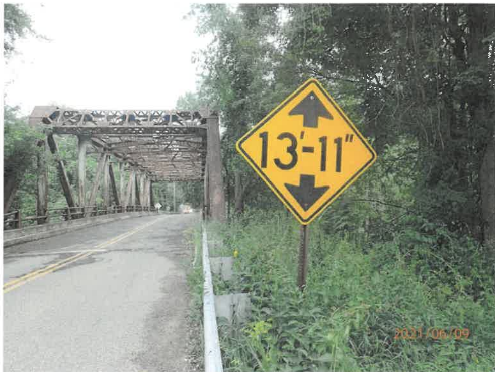
Photo 2: East Approach At-Bridge Clearance Posting
