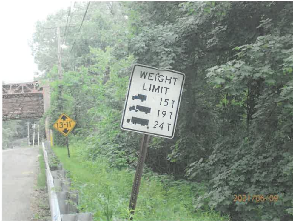
Photo 3: West Approach At-Bridge Weight Posting
