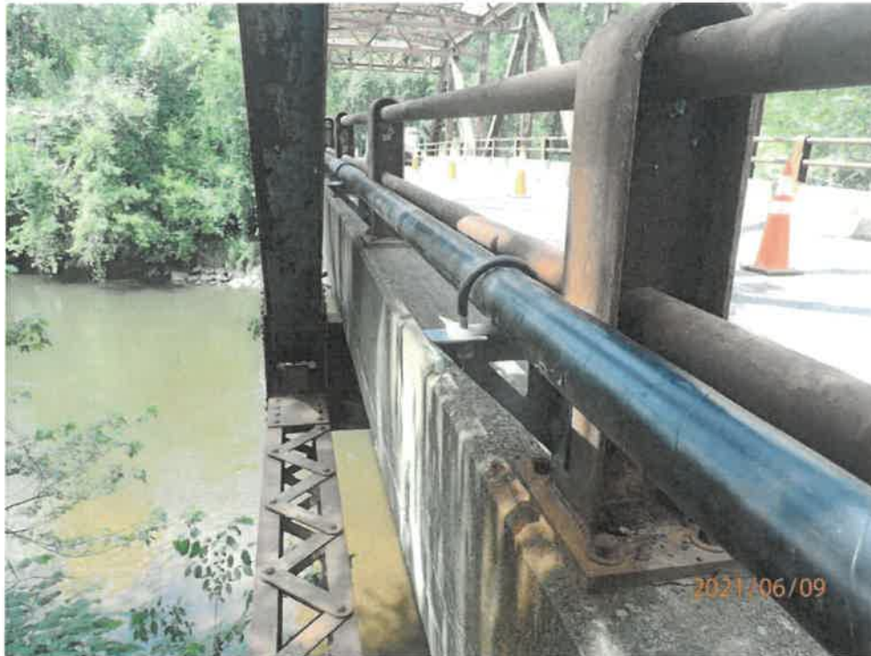
Photo 15: Gas main at South side of bridge
