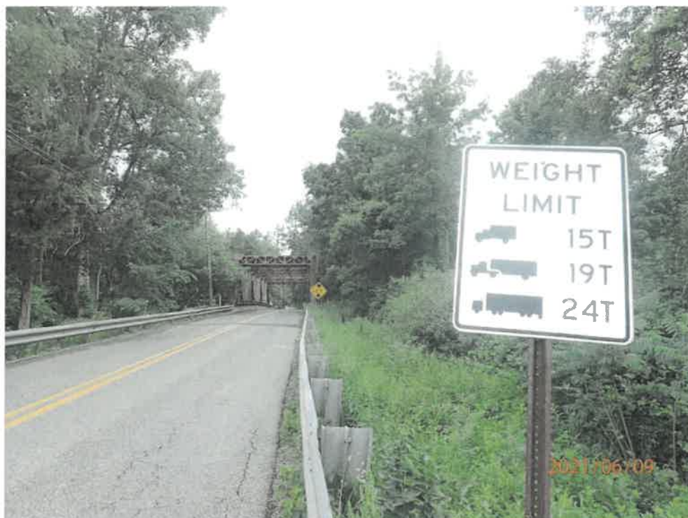
Photo 4: East Approach At-Bridge Weight Posting
