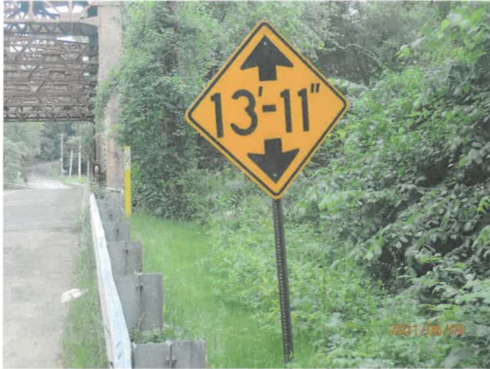
Photo 1: West Approach At-Bridge Clearance Posting
