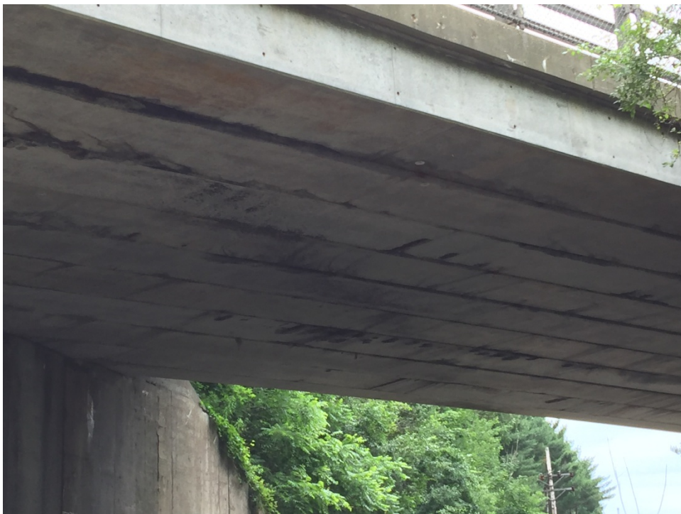
P-10-002 (0DY) UNDERSIDE OVERVIEW
