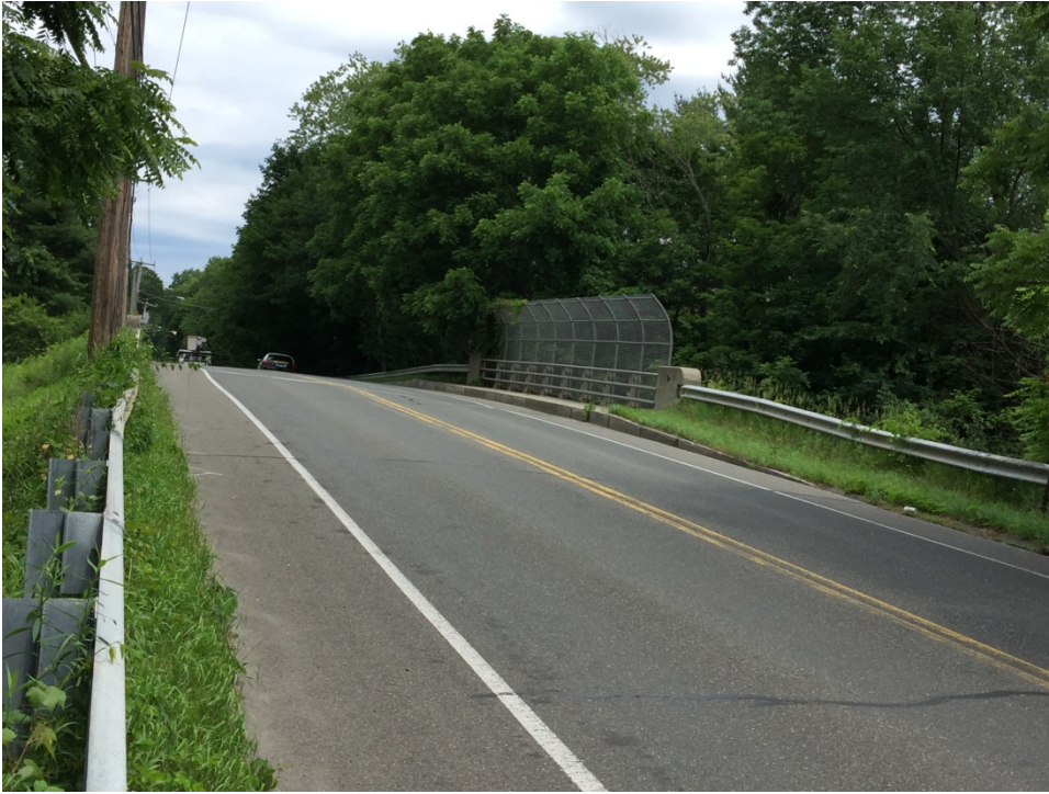
P-10-002 (0DY) WEST APPROACH LOOKING EAST
