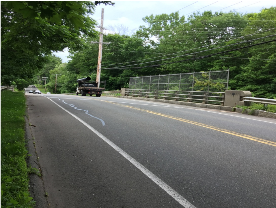
P-10-002 (0DY) EAST APPROACH LOOKING WEST
