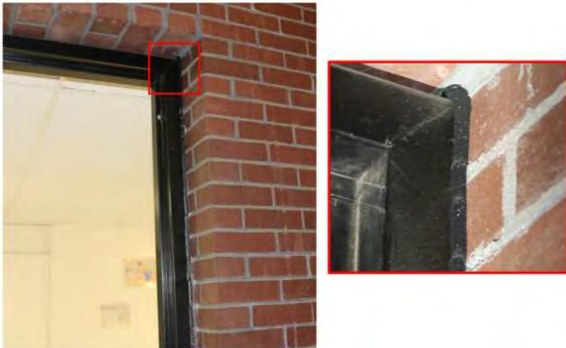
Figure 11. Joint caulk found in room 28 containing 84,500 ppm PCBs.
