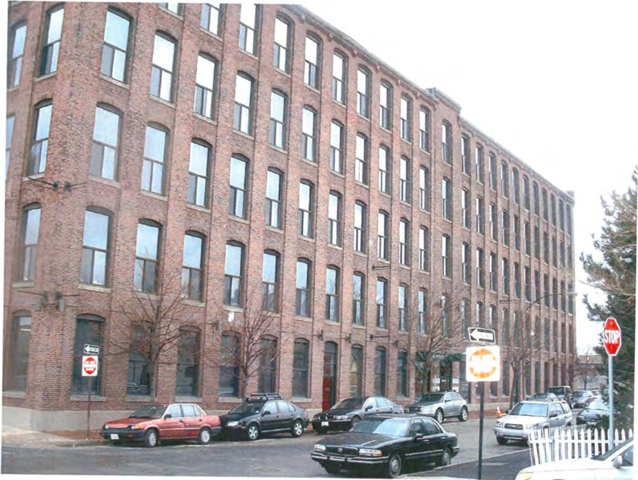
The building was assessed and the exterior envelope was acoustically tested to determine appropriate acoustical treatments. The Foundry's solid brick bearing walls block most outside noise from entering the building, but the existing windows were found to be a significantly weaker sound barrier. All existing windows on the Second through Fifth Floors will be replaced with new dual aluminum acoustical fixed and gliding units. The window installation also
