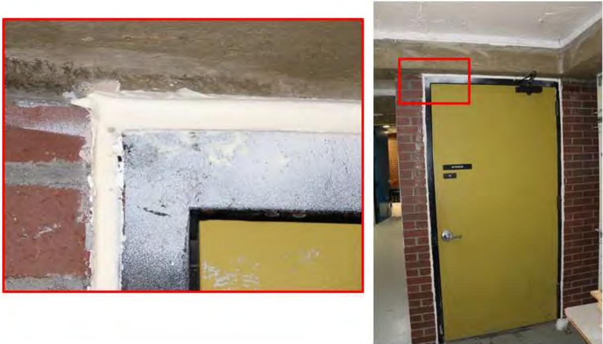
Figure 5. Typical joint sealing caulk found at Westport Middle school located outside storage room 12
