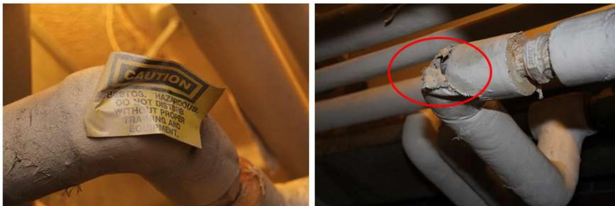
Figure 9. Piping containing asbestos insulation in the gym mechanical room.
