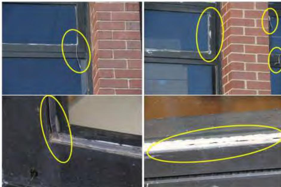
Figure 7. Typical weathered, degraded and non-functioning caulk on the outside of the Westport Middle School. Yellow highlighted areas indicate examples of deteriorated caulk
