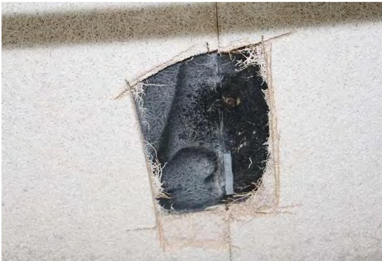
Figure 8. Image of Tectum ceiling panel (white fibrous material) found above drop ceiling in hallway, that has been cut open to expose the underlying felt layer (black material).
