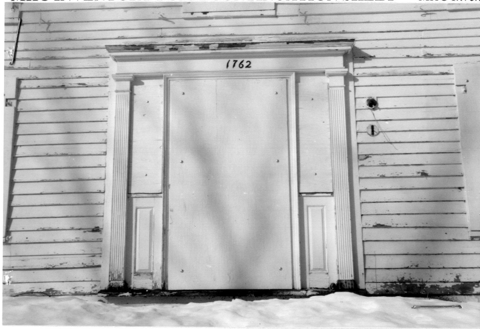
View West, door detail
