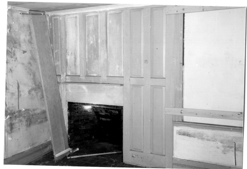
Interior view Northwest in North room, 2 nd Floor
