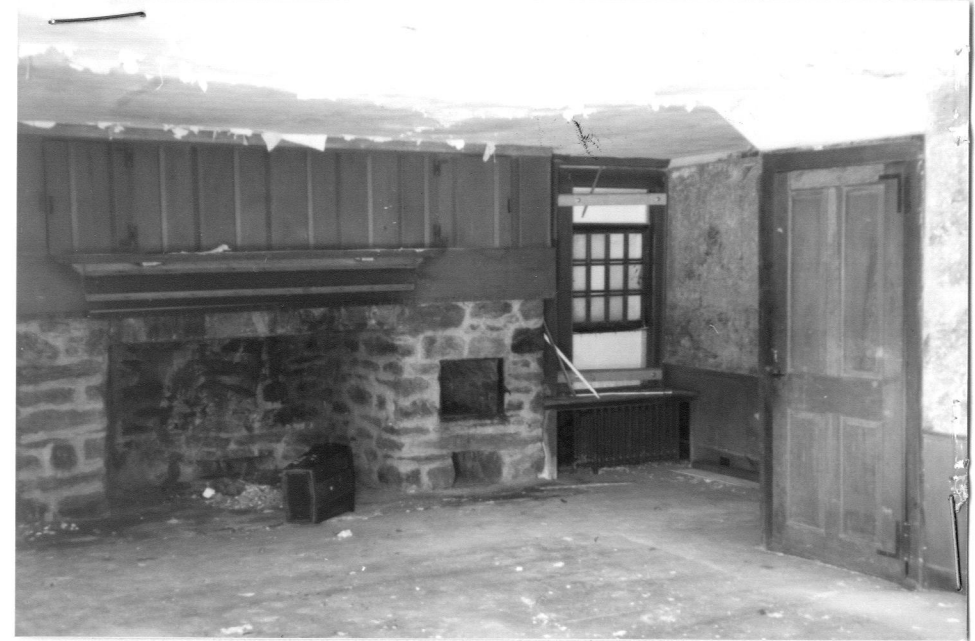
Interior view West in South room, 1 st Floor
