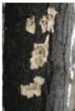
Figure 5. Jagged holes left by woodpeckers.
