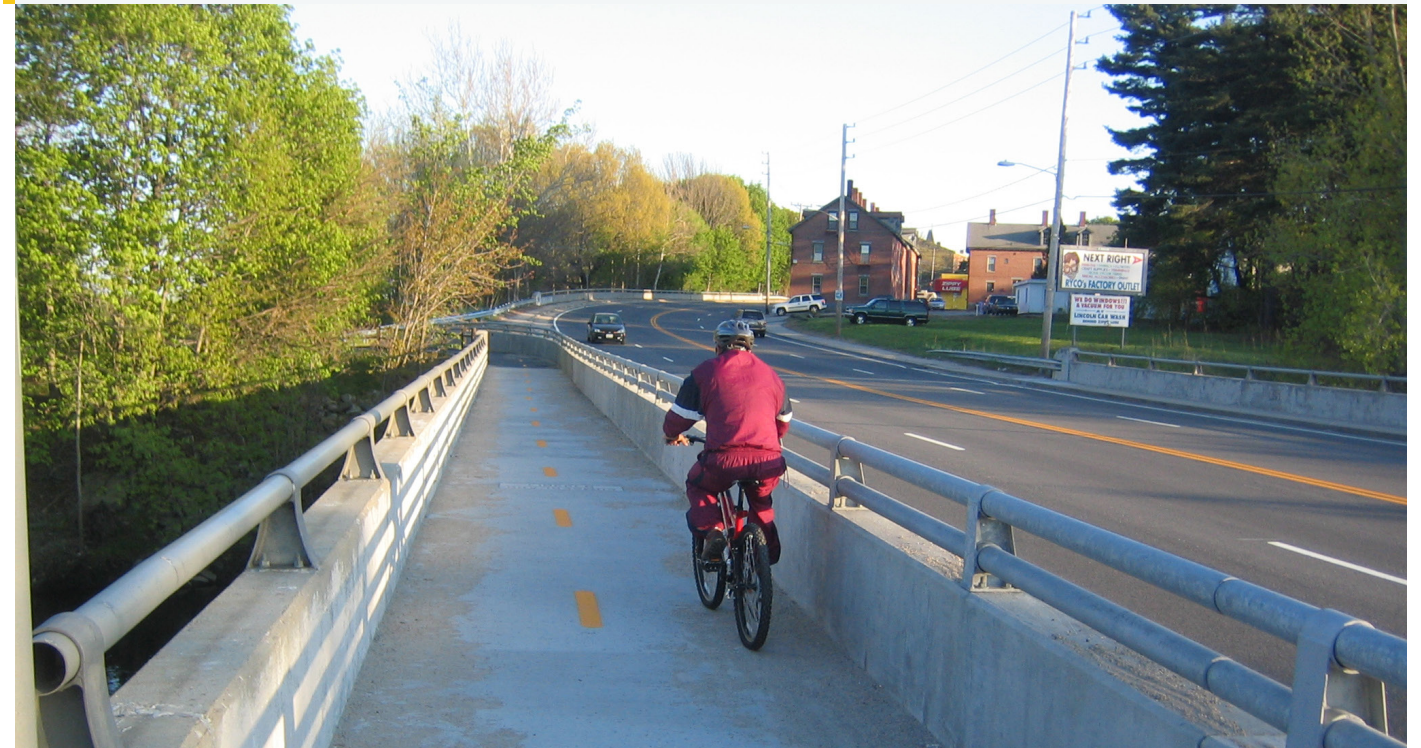
Figure 19 —Bidirectional shared-use path recently installed on a Route 122 bridge in Cumberland, Rhode Island
