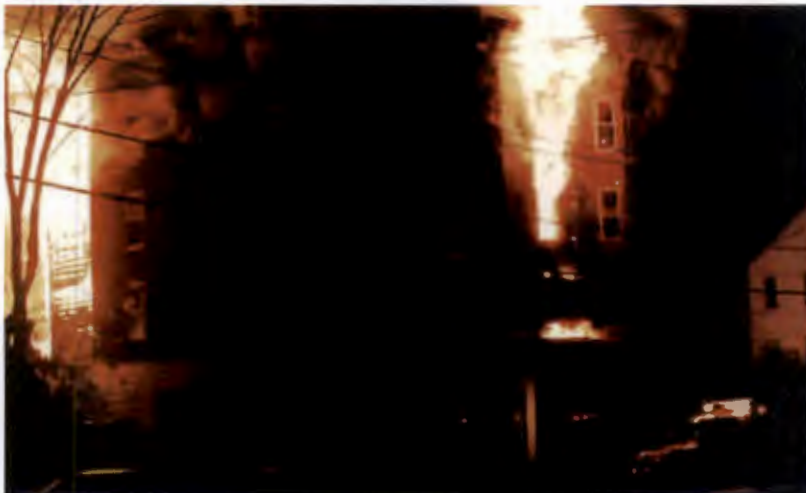
Counter and concurrent flame spread on rear porches
