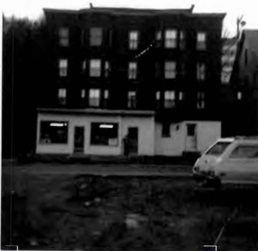
Pre-fire image of "A" side, front of building
