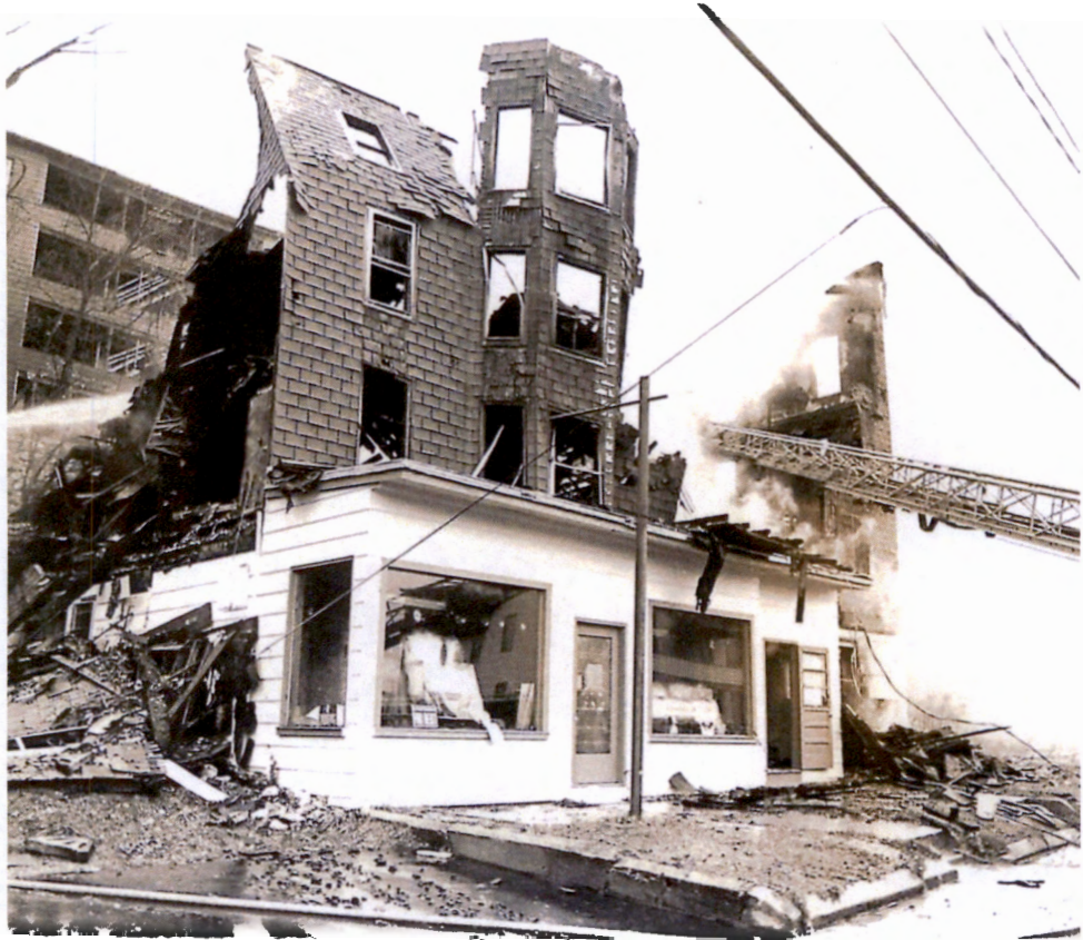
Post fire image of "A," "D" corner
