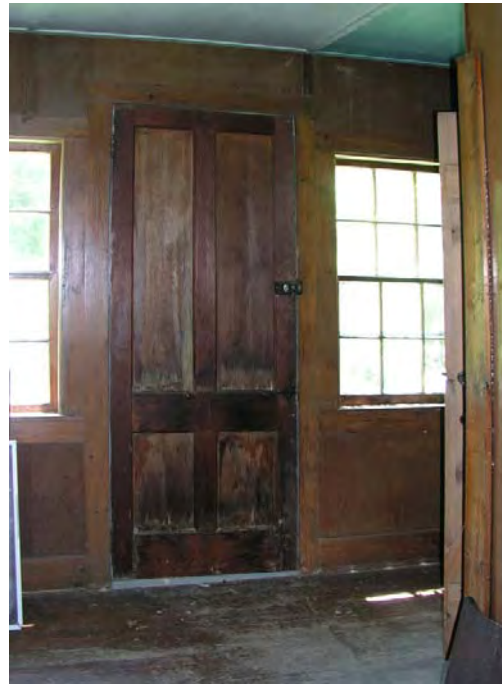
Fig. 5.13. Interior face of recessed-panel door at ell.
