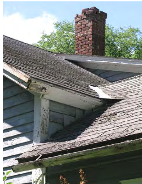
Fig. 5.3. Existing valleys and stepped flashing.
