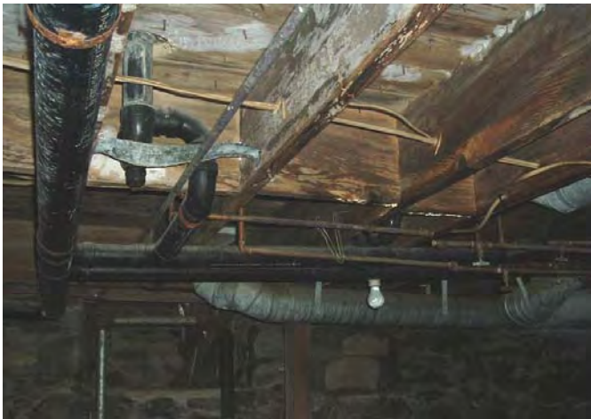
Fig. 4.1. Typical condition, basement ceiling (first-floor framing).
