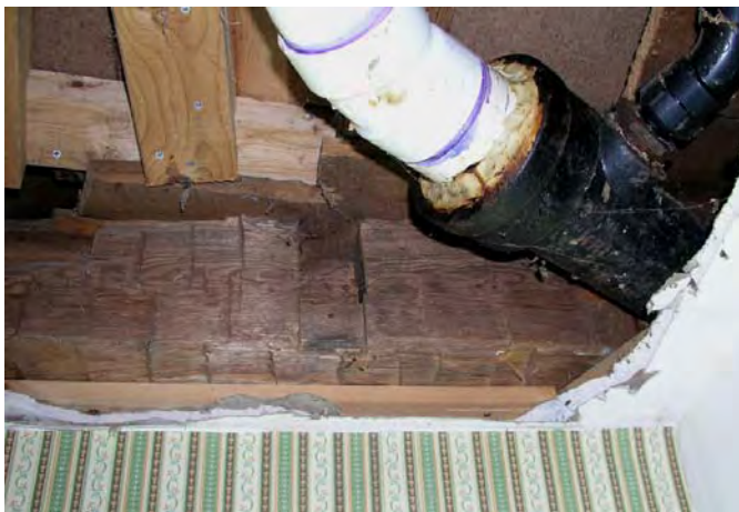
Fig. 6.11. Hand-hewn beam and modern additions.
