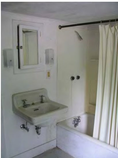
Fig. 4.6. Second-floor bathroom fixtures.
