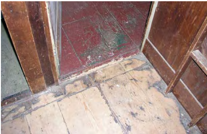
Fig. 6.4. Joints in wide-board pine flooring at second floor seems to indicate prior changes to the floor plan.
