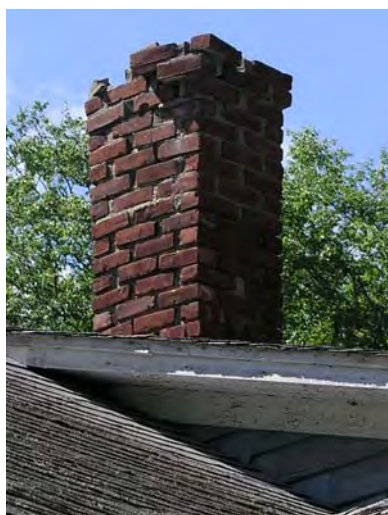
Fig. 5.10. Brick (flue) chimney.
