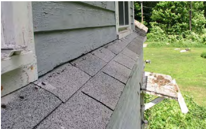
Fig. 5.1. Roof adjacent to east dormer.
