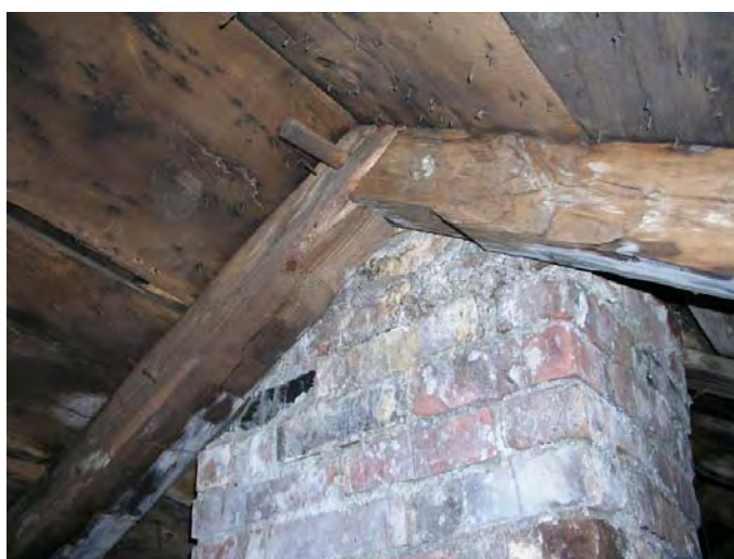
Fig. 5.11. Chimney at attic.
