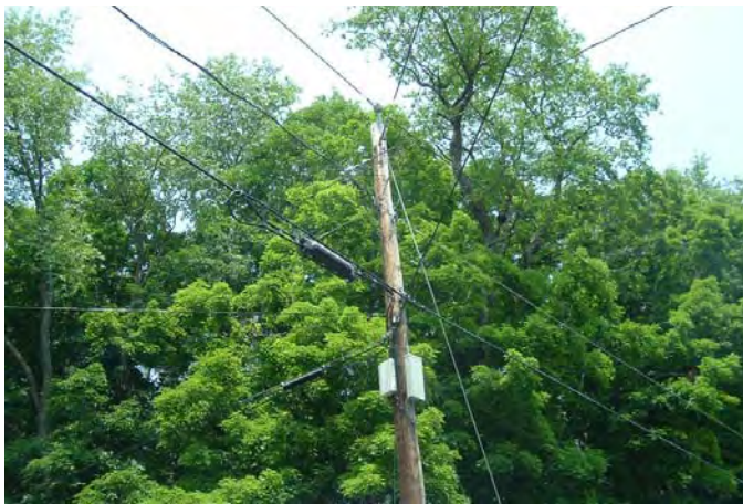
Fig. 4.3. Existing utility pole.
