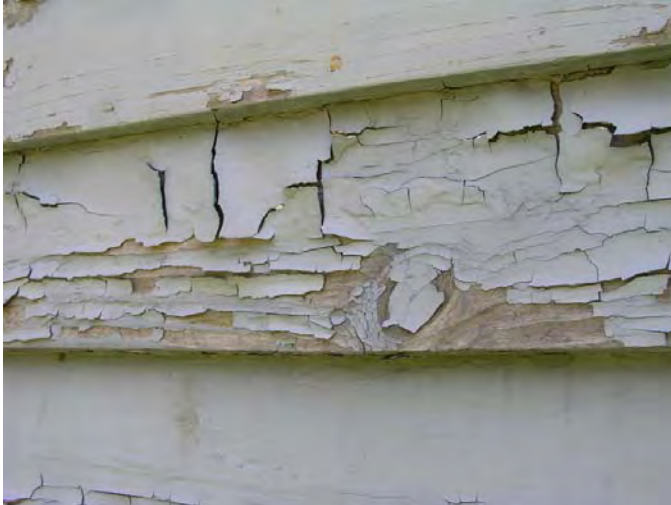
Fig. 5.6. Typical condition at clapboard siding, 2007.
