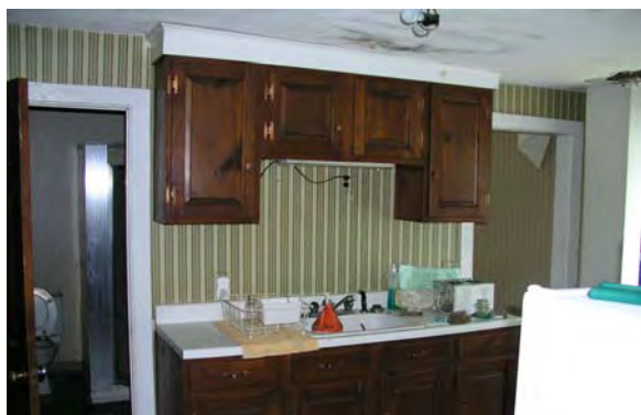
Fig. 6.7. The existing kitchen cabinets and wallpaper.
