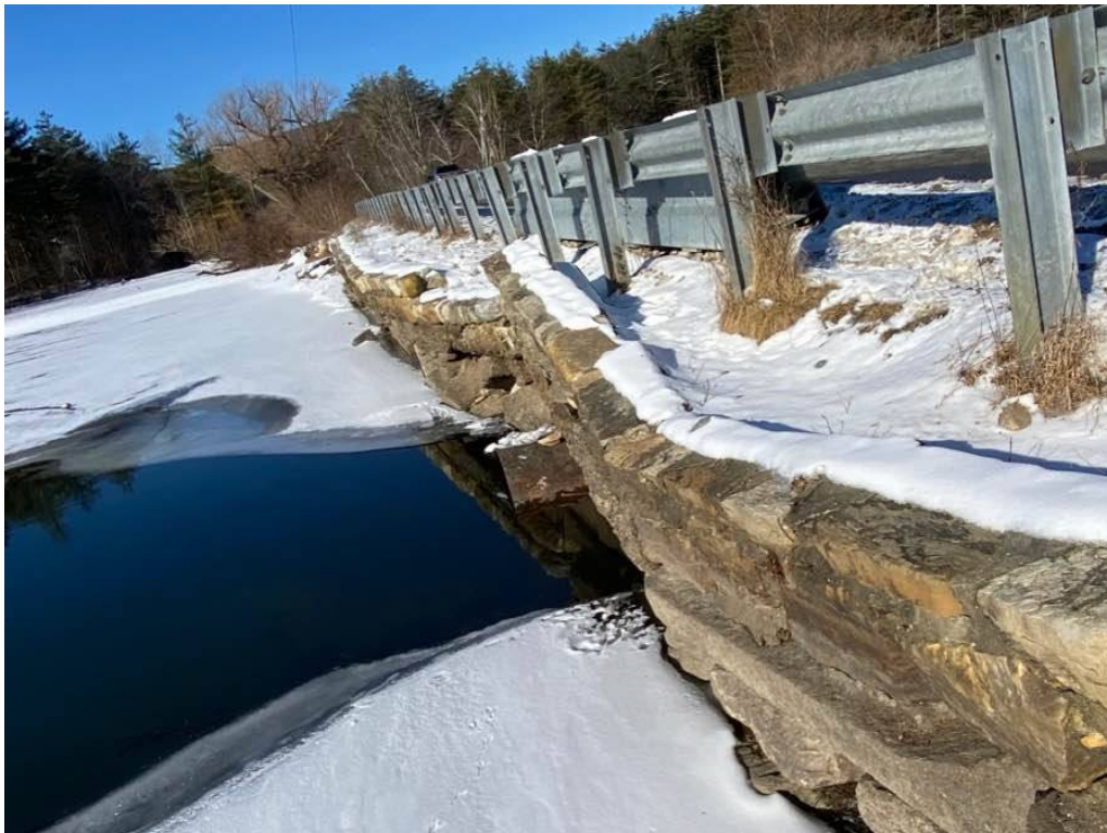
Photo 2: South end of the pipe.
