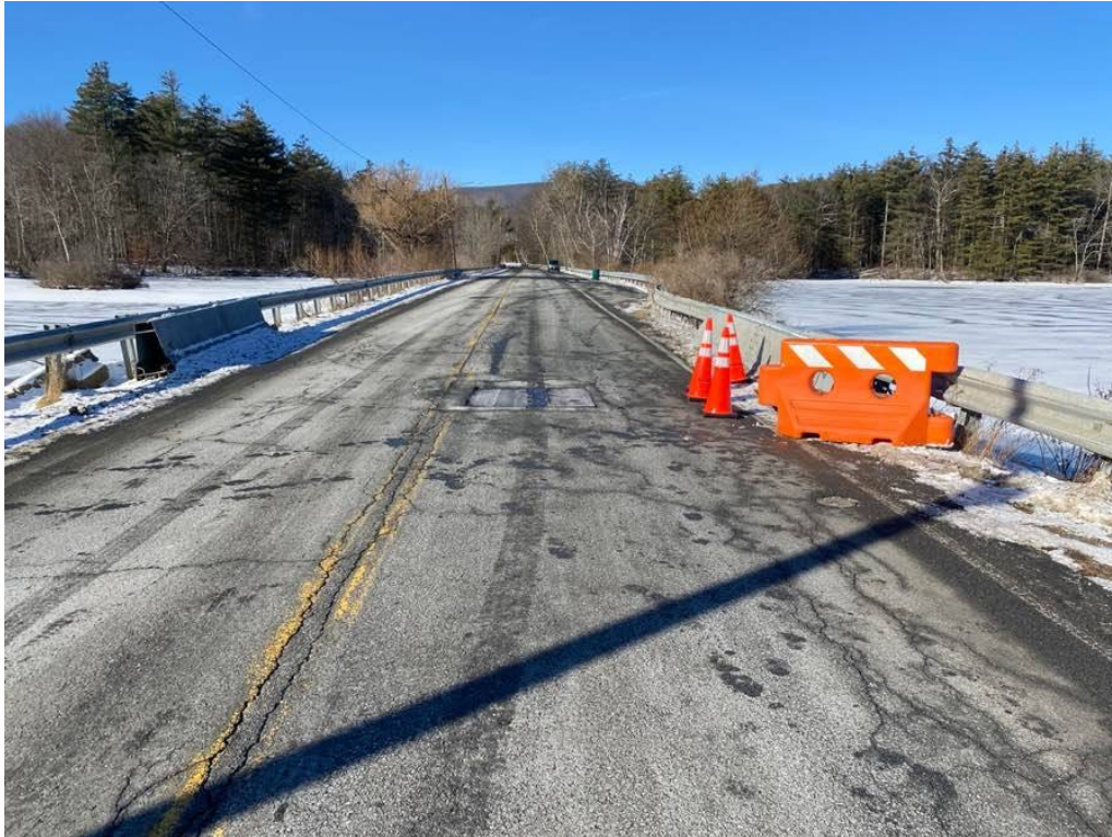
Photo 1: General topside, looking west.
