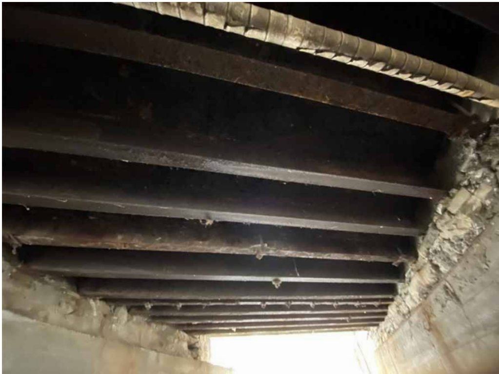
Photo 2: General underside, looking west.
