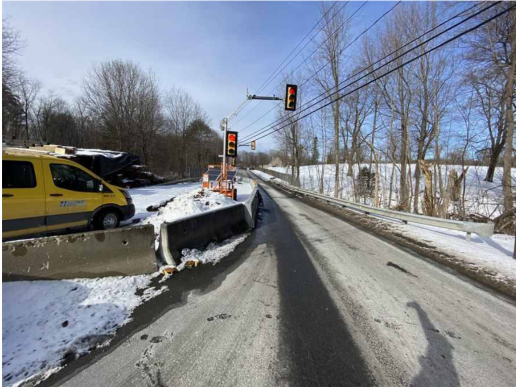
Photo 1: General topside, looking north.
