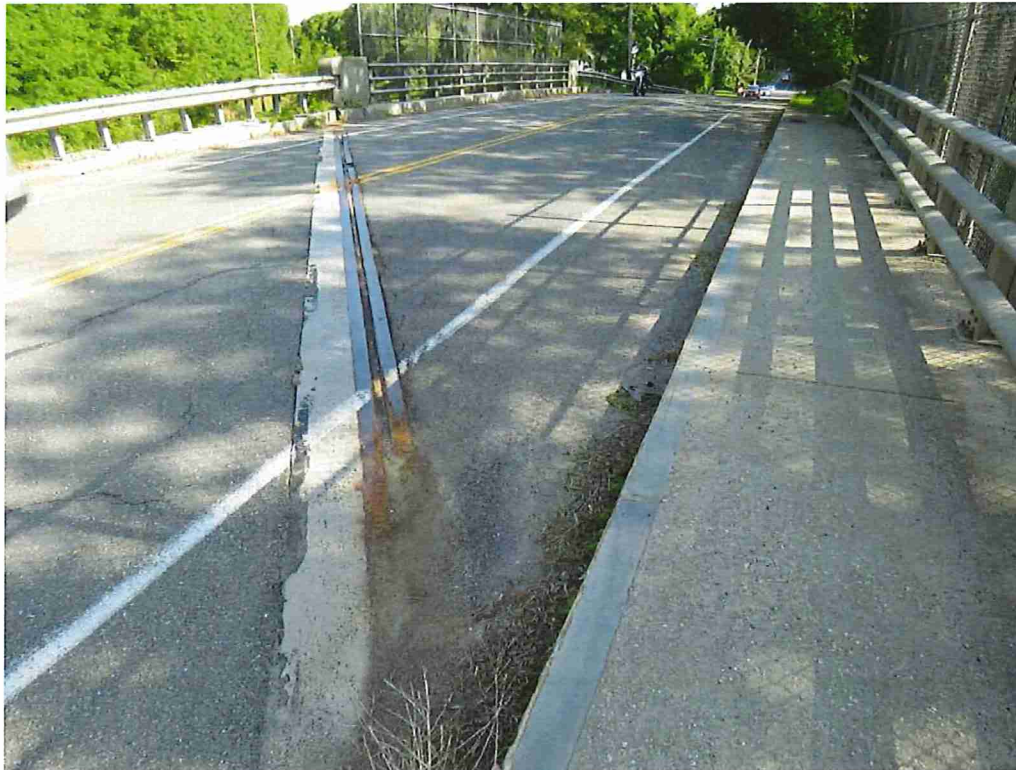
Photo 1: General topside, looking east.
