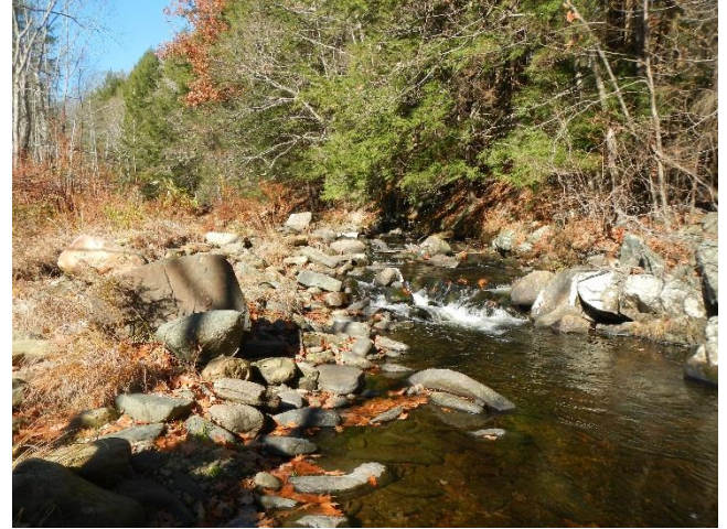
Figure 4.7: Grade controls in reach M05.
