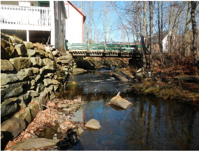
Figure 4.10: Extreme bank armoring on reach M06.B.
