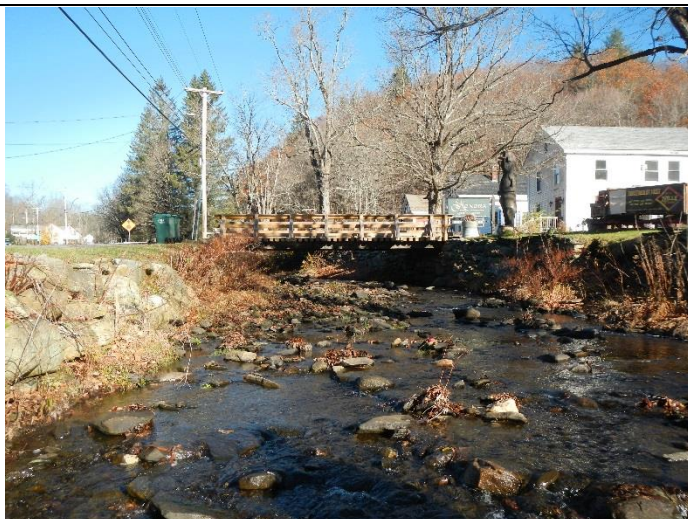
F-type channel due to straightening and armoring.
