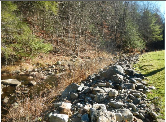
Bank straightening and armoring along cow pasture.
