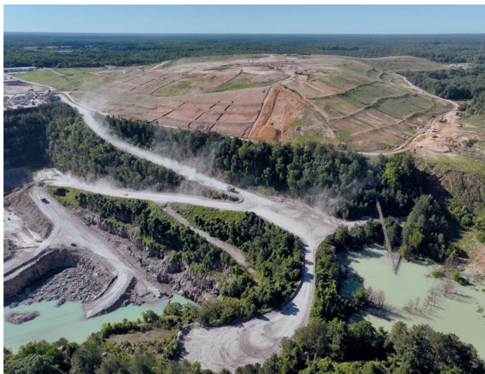
The earthen mound at the top of this photo is the Shoosmith Landfill near Richmond. The landfill sought unsuccessfully to expand into the quarry in the foreground. (Courtesy of Chesterfield County, VA)
