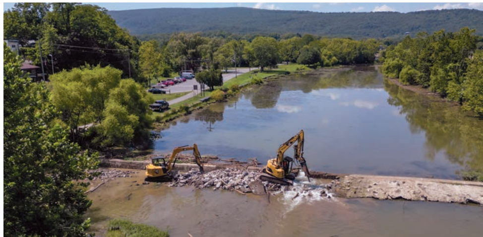
Rock breakers work to remove an obsolete dam across the Raystown Branch of the Juniata River in Bedford, PA, in August 2025. (Matt Otis)
