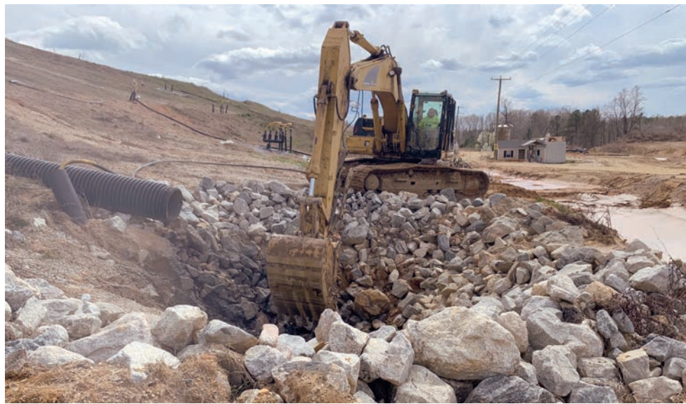
A worker at the at the Shoosmith Landfill uses an excavator to replace riprap around a stormwater "drop inlet" in March 2024. (Bruce Coble)
