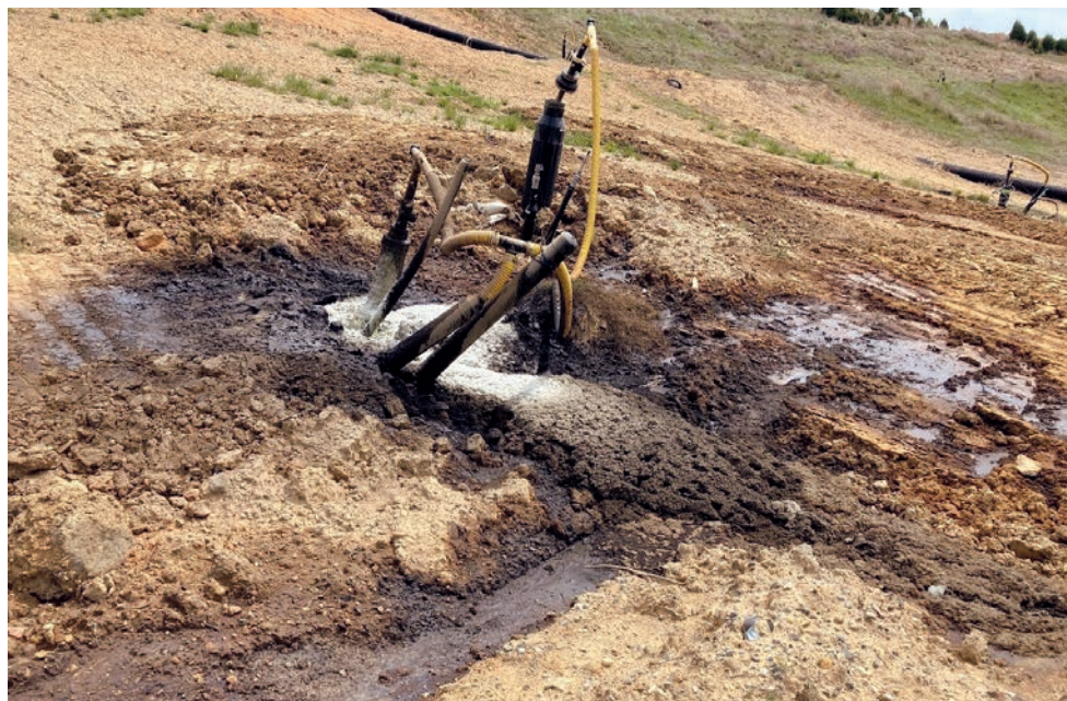
Leachate can be seen percolating to the surface at the Shoosmith Landfill in this April 2026 photo provided by the Virginia Department of Environmental Quality.
