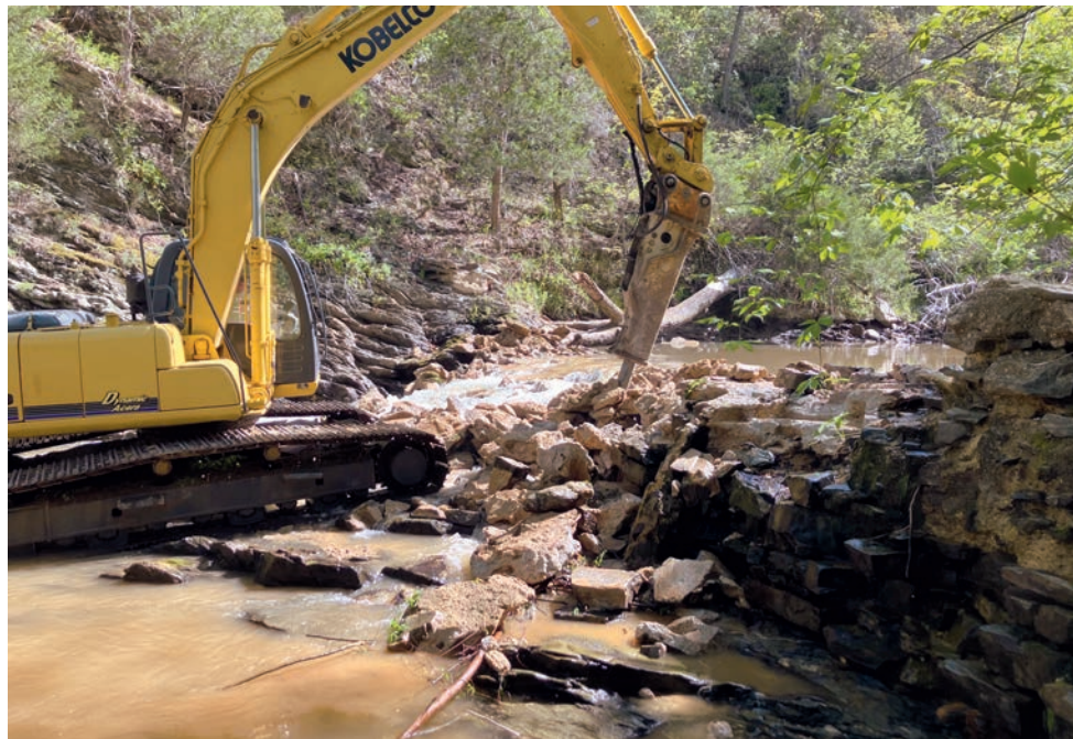
A hydraulic breaker hammers away at the centuries-old Baber’s Mill Dam on Rock Island Creek in Buckingham County, VA, in 2024. (Louise Finger/VA Dept. of Wildlife Resources)
