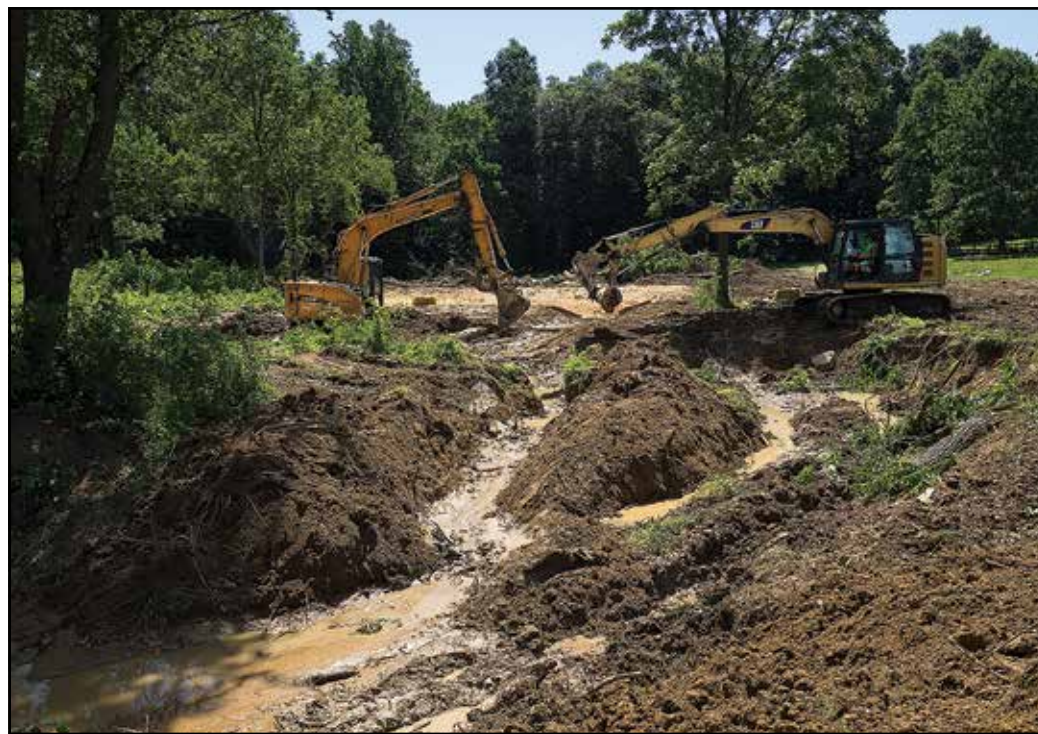
Two excavators work together to carve a new, more stable channel for a tributary of Little Elk Creek in Cecil County, MD. The trunks of streamside trees that have to be removed to refashion the creek channel get used to help stabilize the banks, while their stumps and roots go back in the stream to provide habitat for fish and wildlife. (Dave Harp)
