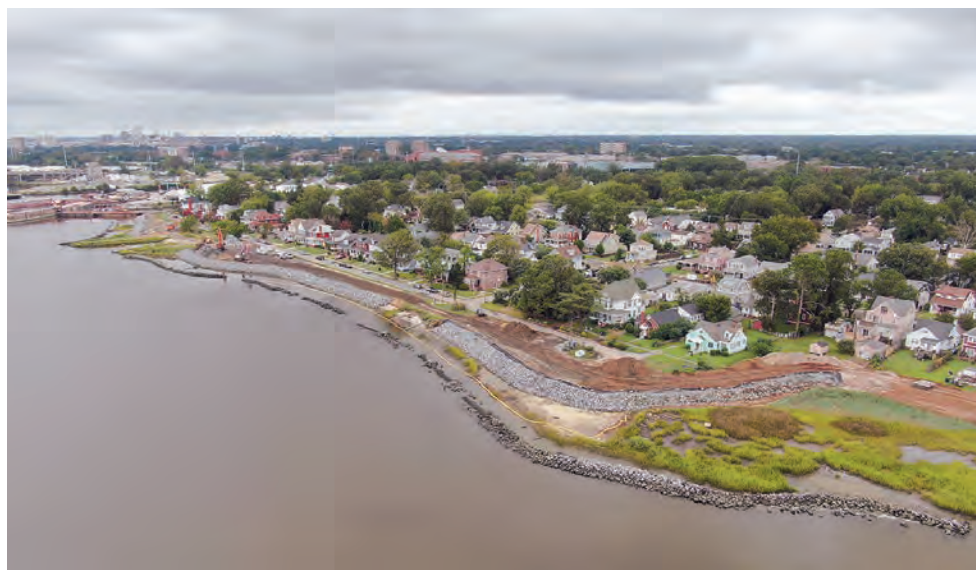
A floodwall is being built to shield the Chesterfield Heights and Grandy Village neighborhoods from tidal flooding along the Elizabeth River's Eastern Branch as part of a "resilience" project largely funded by a $112 million federal grant. (Courtesy of the city of Norfolk)
