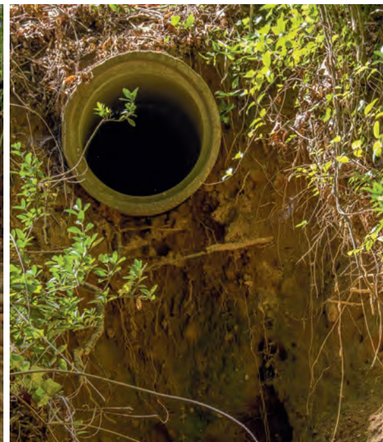
The bank is eroding beneath this stormwater outfall that funnels runoff from homes and pavement into a stream in Goodman Park in Hollin Hills. (Dave Harp)
