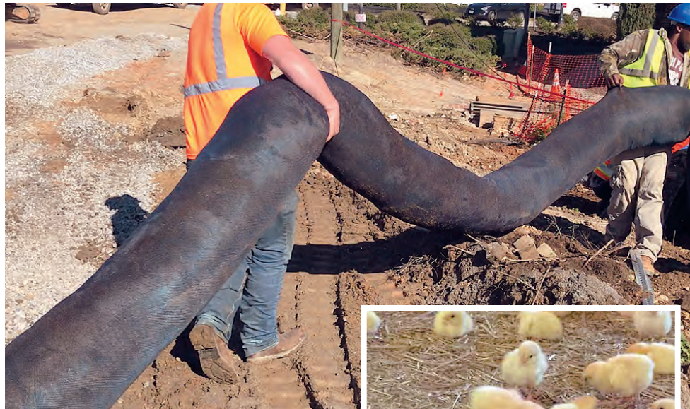
Switchgrass can serve as filling in the erosion control silt socks used at construction sites and for bedding in poultry houses. (Top: MKB Company / Bottom: Association of Warm Season Grass Producers)
