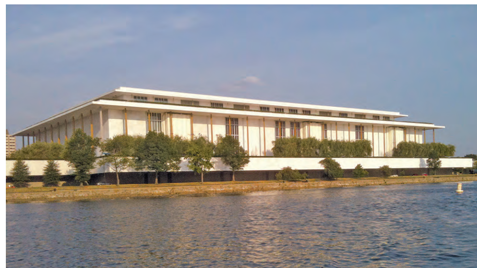
The John F. Kennedy Center for the Performing Arts, shown here from the Potomac River, has settled alleged violations of the Clean Water Act at its facility. (Tom/CC BY 3.0)
