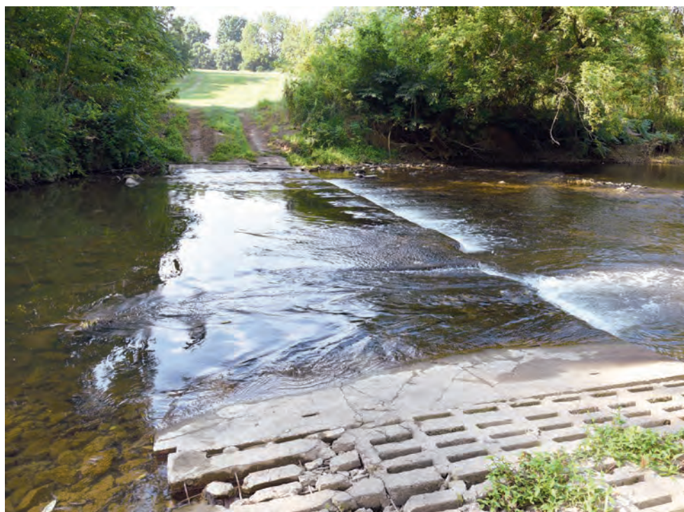
A stream crossing on leased farmland in Pennsylvania helps cows and equipment pass through without causing erosion. (Ad Crable)
