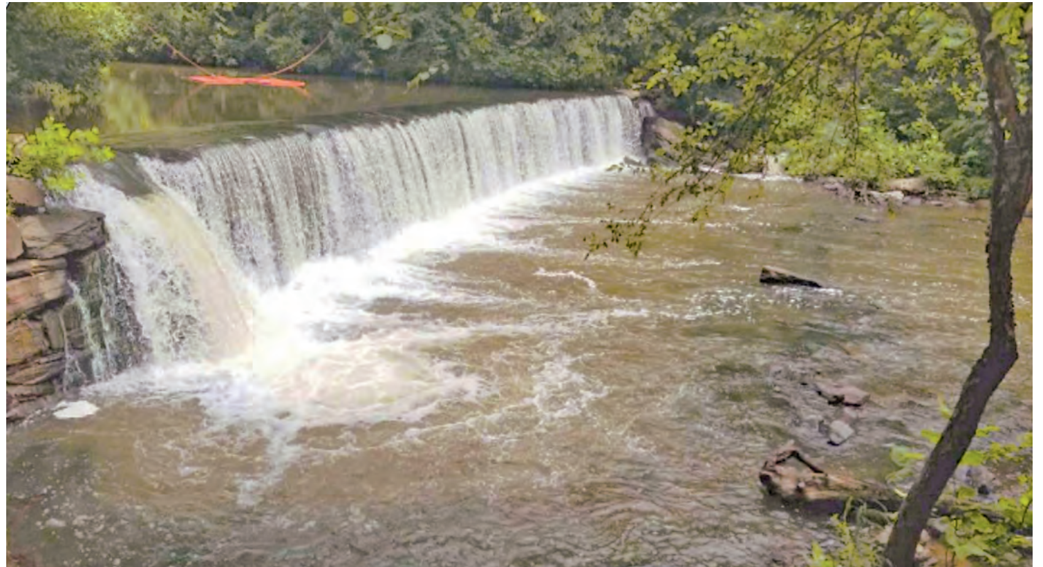
The Jefferson Mill dam was built in 1820 near Charlottesville, VA. Private owners of the site plan to convert the old mill building into a residence and repower the dam to produce energy for the home, while installing a fish passage ramp that will help move migrating fish upstream. (Courtesy of Natel Energy)
