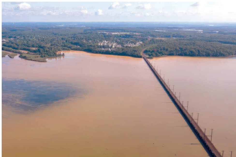
In August 2022, a plume of orange, silt-laden water covers much of Maryland's lower Gunpowder River past the Amtrak rail bridge. (Submitted Photo)
