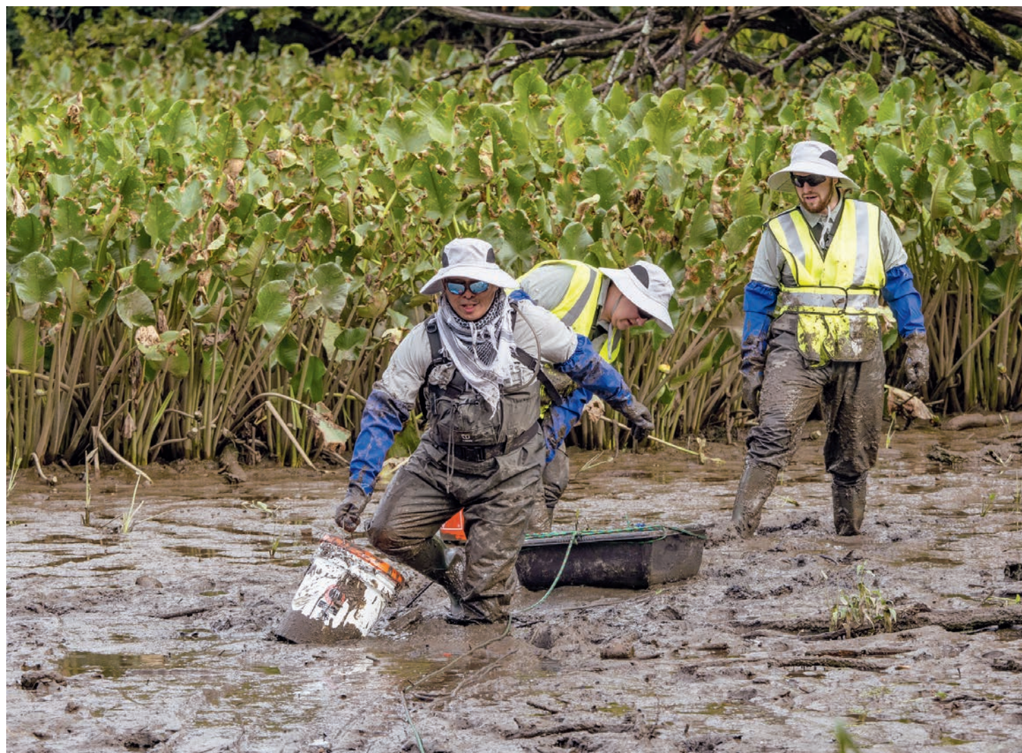
Workers with the Florida-based company ecoSPEARS remove dozens of footlong plastic spears from a cove in the Anacostia River on Aug. 8. Called "spears," after the acronym for their technical name, they spent a year in the sediment, absorbing toxic PCBs as part of an effort to remove them from the local ecosystem. (Dave Harp)
