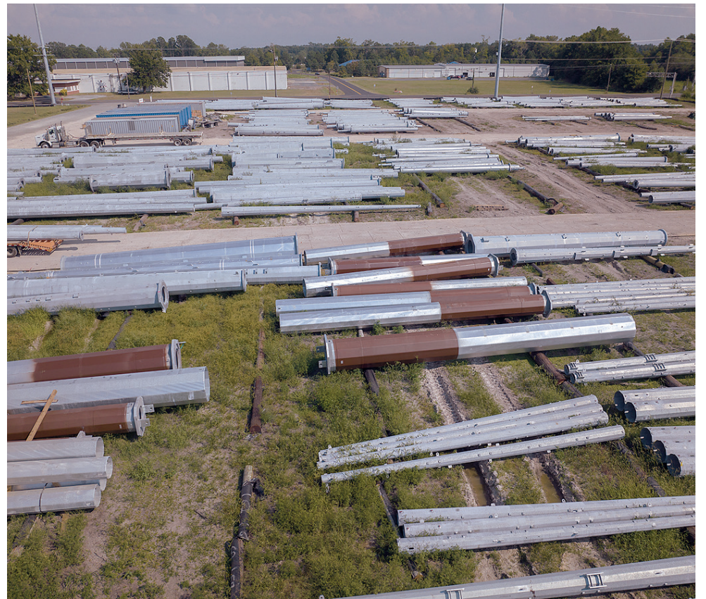
Sections of electric towers lay in a staging yard operated by AUI Power in Cambridge, MD. They will be used for a power line project between Cambridge and the town of Vienna, about 15 miles away. (Dave Harp)
