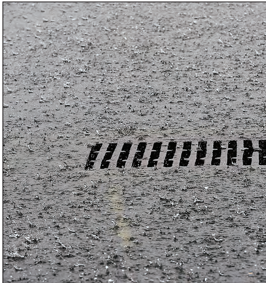
One inch of rain on just one acre of hardened surface produces about 27,000 gallons of polluted runoff. (Dave Harp)
