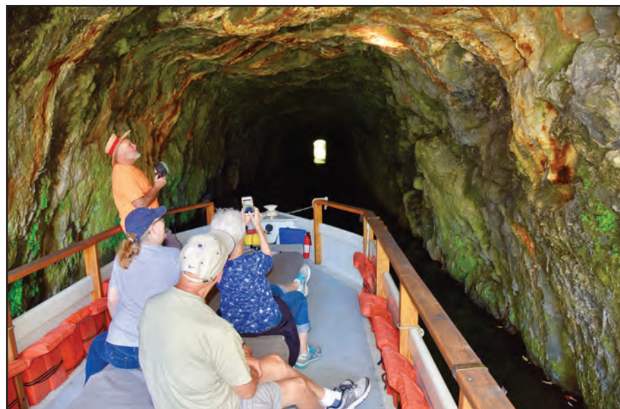
Workers hand-cut stone in the 1820s to forge this tunnel on the Union Canal, built to connect commerce between Philadelphia on the Schuylkill River and Harrisburg along the Susquehanna. (Ad Crable)
