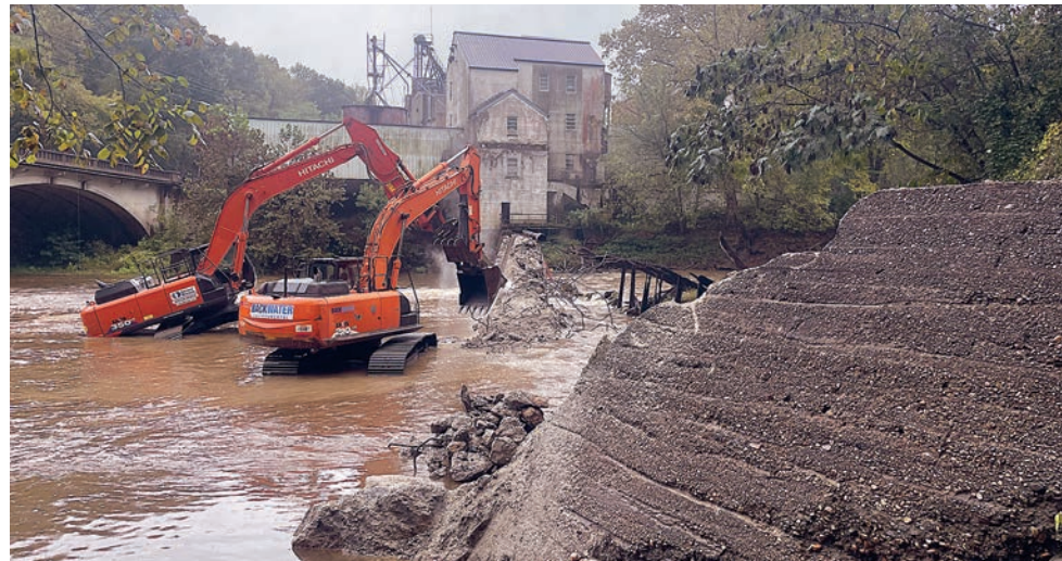
Excavators demolish a dam on the South Anna River in Ashland, VA, on Oct. 1. Removing the dam gives migratory of fish access to more than 400 miles of historic spawning grounds. (Whitney Pipkin)
