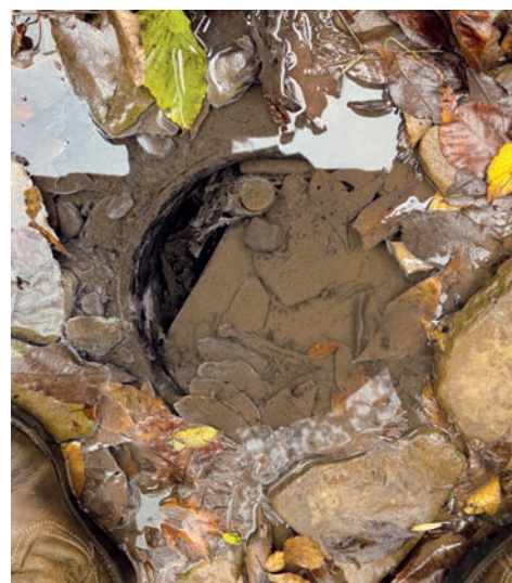
Methane and arsenic leak from the metal casing of an abandoned wellhead in Pennsylvania. (Ad Crable)
