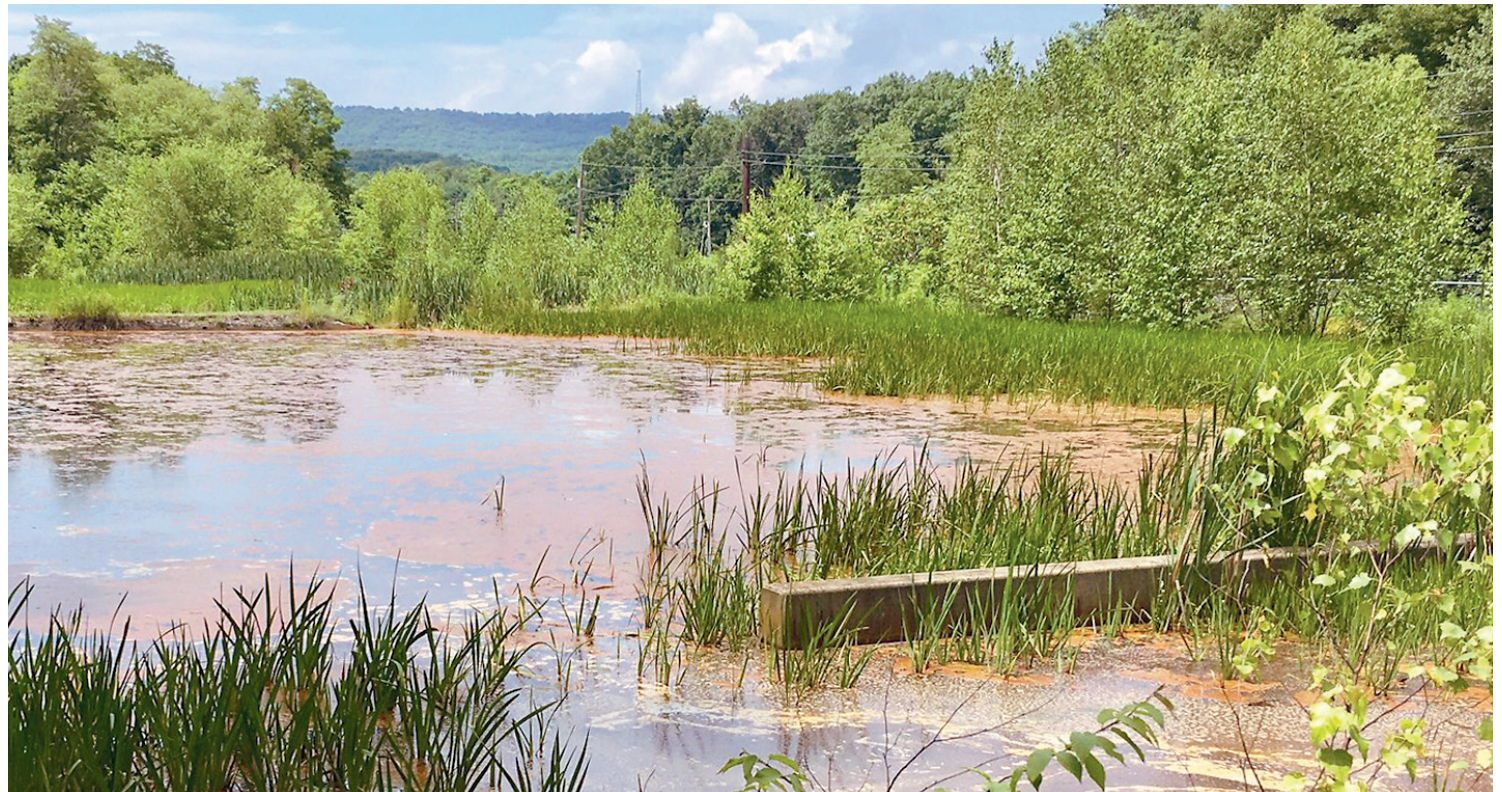
A constructed wetland in Pennsylvania provides a place where plants and bacteria remove heavy metals and acidity from mine drainage. (Earth Conservancy)
