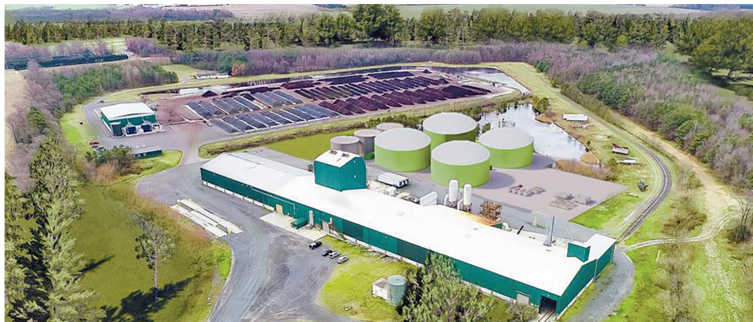
A rendering of the proposed anaerobic digester near Seaford, DE, shows new tanks where waste will be broken down to create biogas. The existing building in the foreground, Perdue’s former pellet fertilizer plant, will house other components of the digester. The composting facility is in the background. (Bioenergy DevCo)
