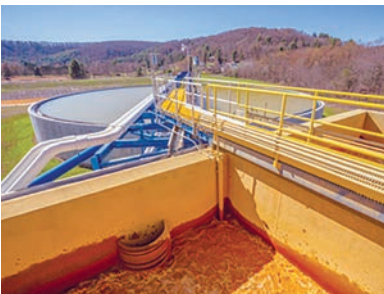
A $2.1 million treatment plant on 41 acres removes heavy metals and acidity from 20 discharge points of acid mine drainage in northwestern Pennsylvania. See story on page 20. (West Branch Susquehanna Restoration Coalition)
