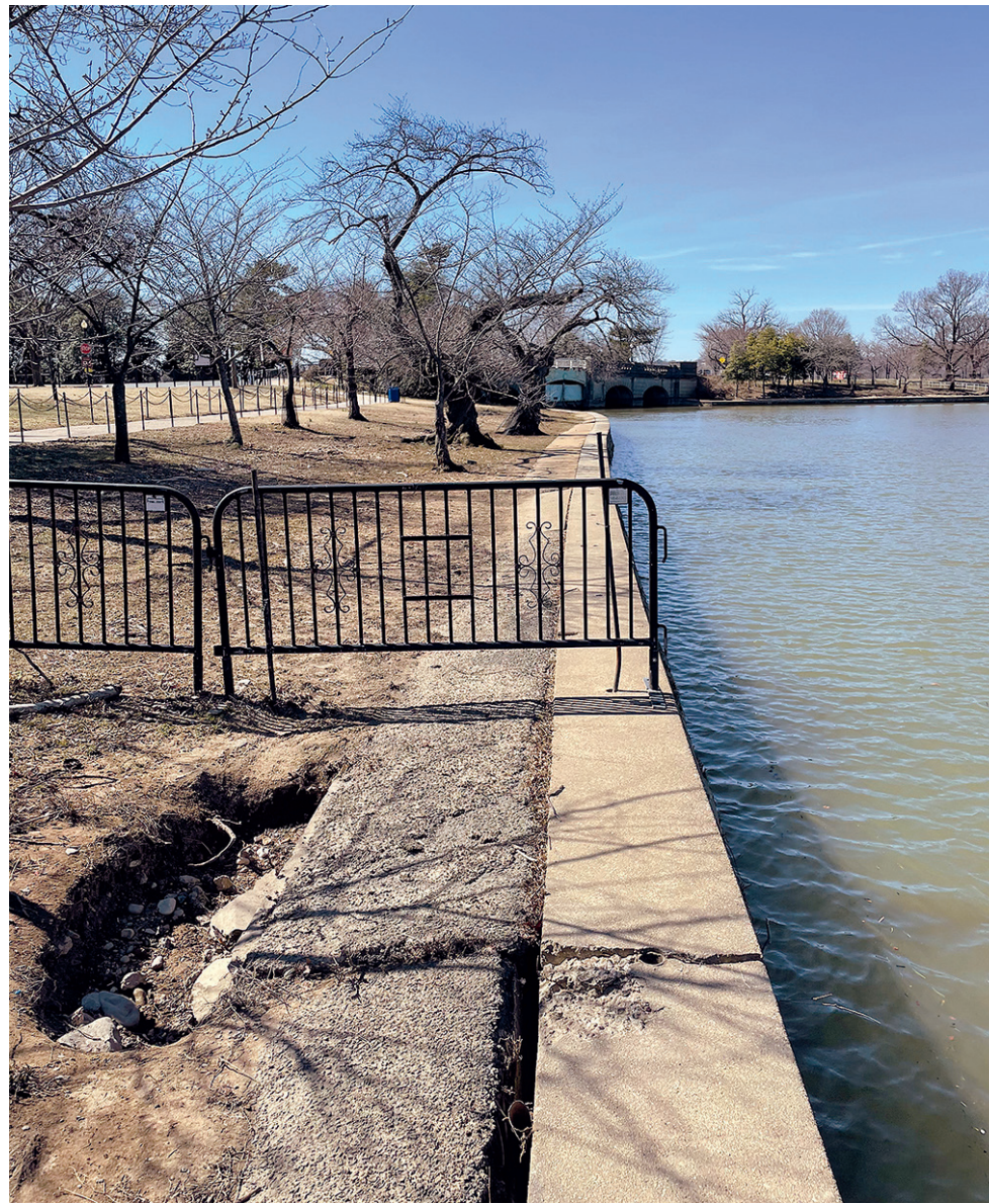
Rising tides overwhelm portions of the seawall twice daily at the Tidal Basin, leaving holes and crumbling pavement in their wake. (Whitney Pipkin)
