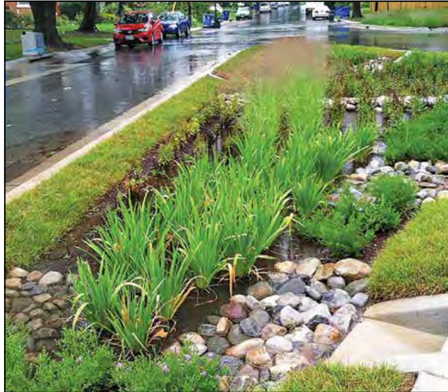
Rain gardens, bioswales and other green infrastructure, like this one on a residential Montgomery County street corner, capture runoff and reduce the flow of nutrient-laden stormwater to local streams. Environmental groups worry that as the county looks to cut costs, streams might suffer if small projects like this get dropped. (Montgomery County MD Department of Environmental Protection)
