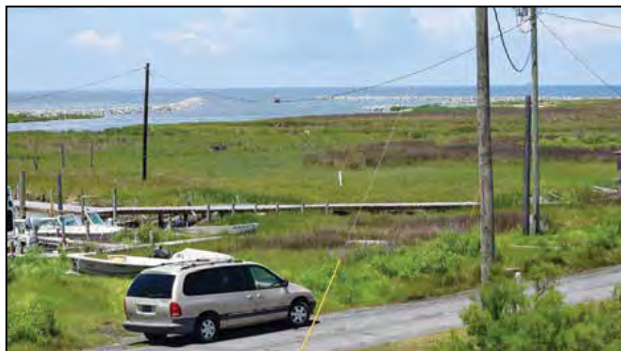
Two jetties extending out into the Bay were built by the U.S. Army Corps of Engineers to protect a navigational channel near Rhodes Point on Smith Island. (Jeremy Cox)
