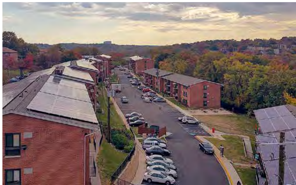
DC's Solar for All program, which aims to bring cheaper solar electricity to low-income households, resulted in this community solar array on roofs at the Atlantic Terrace Apartments in 2018. (WinnCos)
