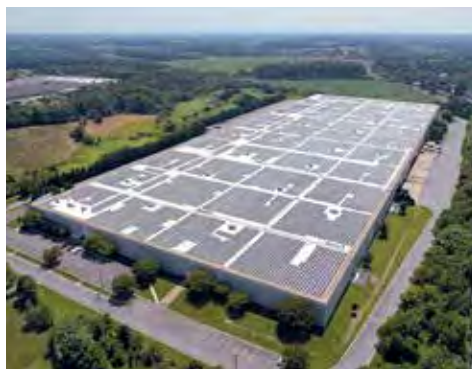
This community solar array atop a warehouse in Carroll County, MD, has attracted 1,300 nearby residential and commercial subscribers, saving them money on future electric bills. One-third are low- and moderate-income residents. (Summit Ridge Energy)
