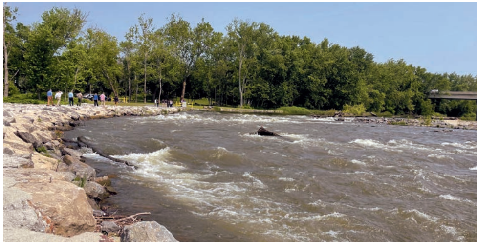
The $5.3 million fish passage at Shikellamy State Park mimics a natural channel by creating pools and riffles that are suitable for a variety of fish species. (Karl Blankenship)
