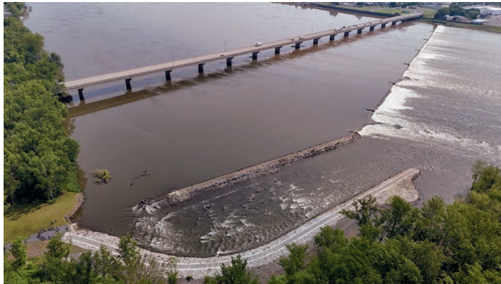
A 900-foot-long fish passage at Shikellamy State Park in Pennsylvania bypasses the inflatable dam that has blocked the Susquehanna River every summer since 1969. (Commonwealth Media Services)
