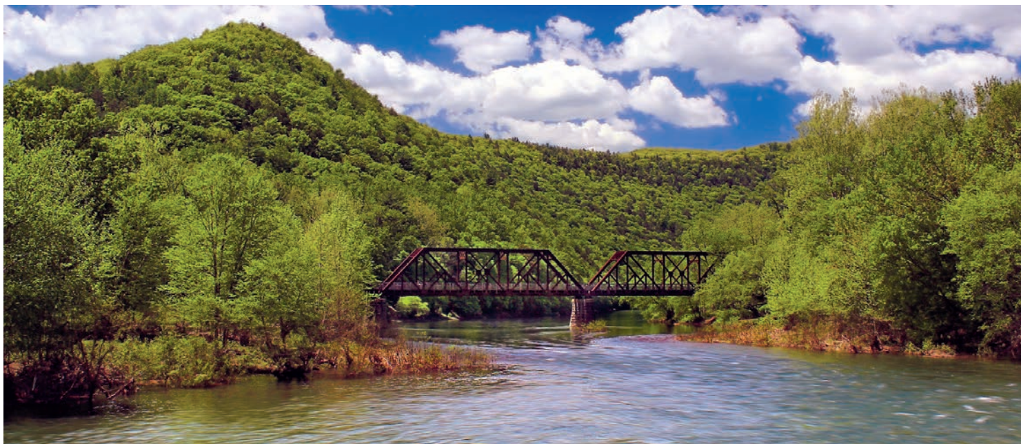
An iron bridge carries the rail trail over Pine Creek near Tiadaghton State Forest in Lycoming County, PA. (Nicholas A. Tonelli/CC BY 2.0)
