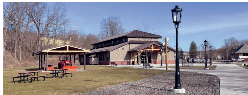
The Patterson Trailhead Building, a welcome center, stands ready for visitors to the three-mile extension of the trail. (Carolyn Beans)
