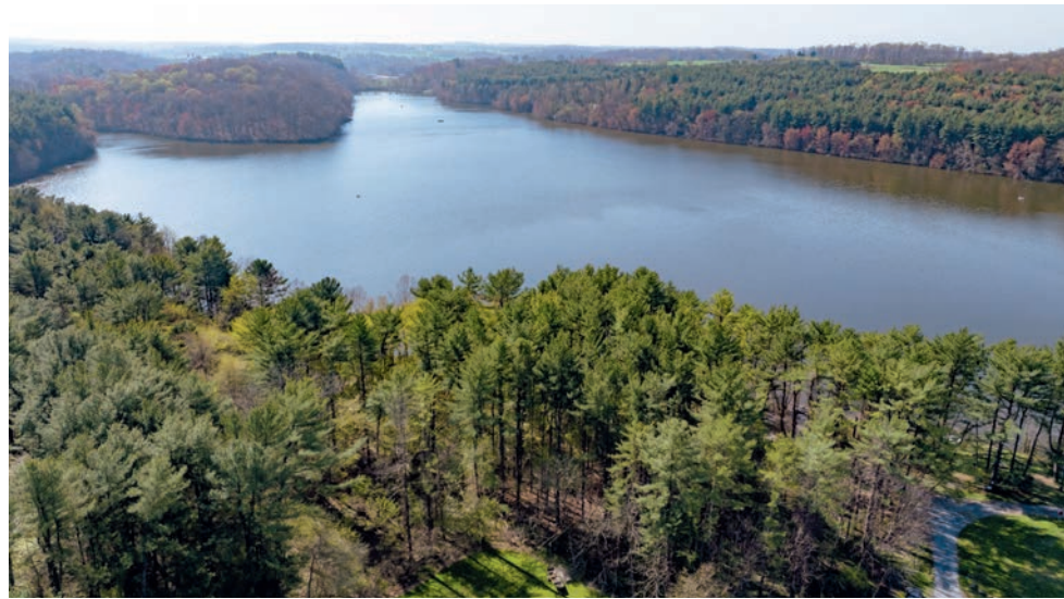
The Octoraro Reservoir in southeastern Pennsylvania was created by a dam built in the 1950s on Octoraro Creek, a tributary of the Susquehanna River. (Dave Harp)
