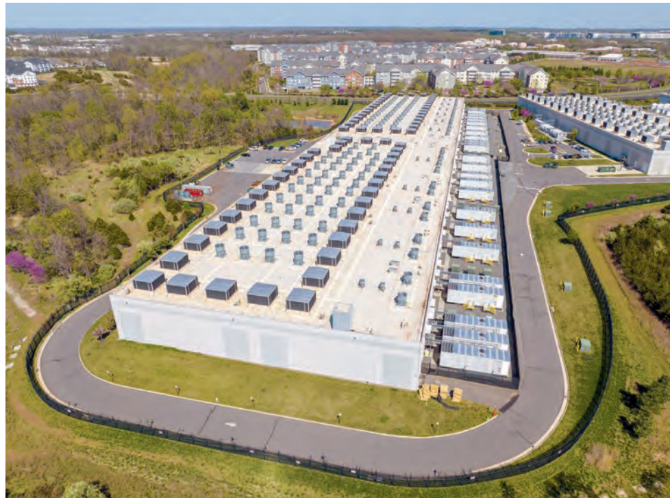
Tractor trailer-size generators run the entire length of a data center building in Loudoun County, VA. (Hugh Kenny/Piedmont Environmental Council)
