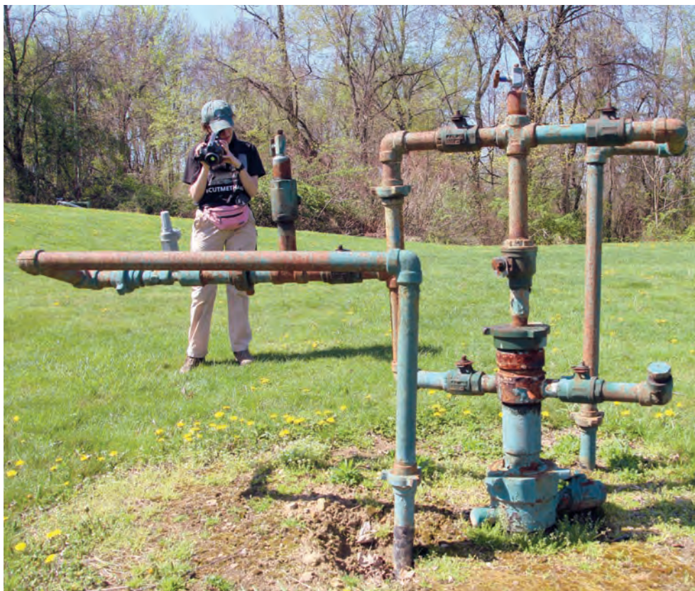
Melissa Ostroff, a licensed thermographer for the environmental group Earthworks, used an infrared camera to detect methane leaks from a natural gas well in Pennsylvania. (Earthworks)
