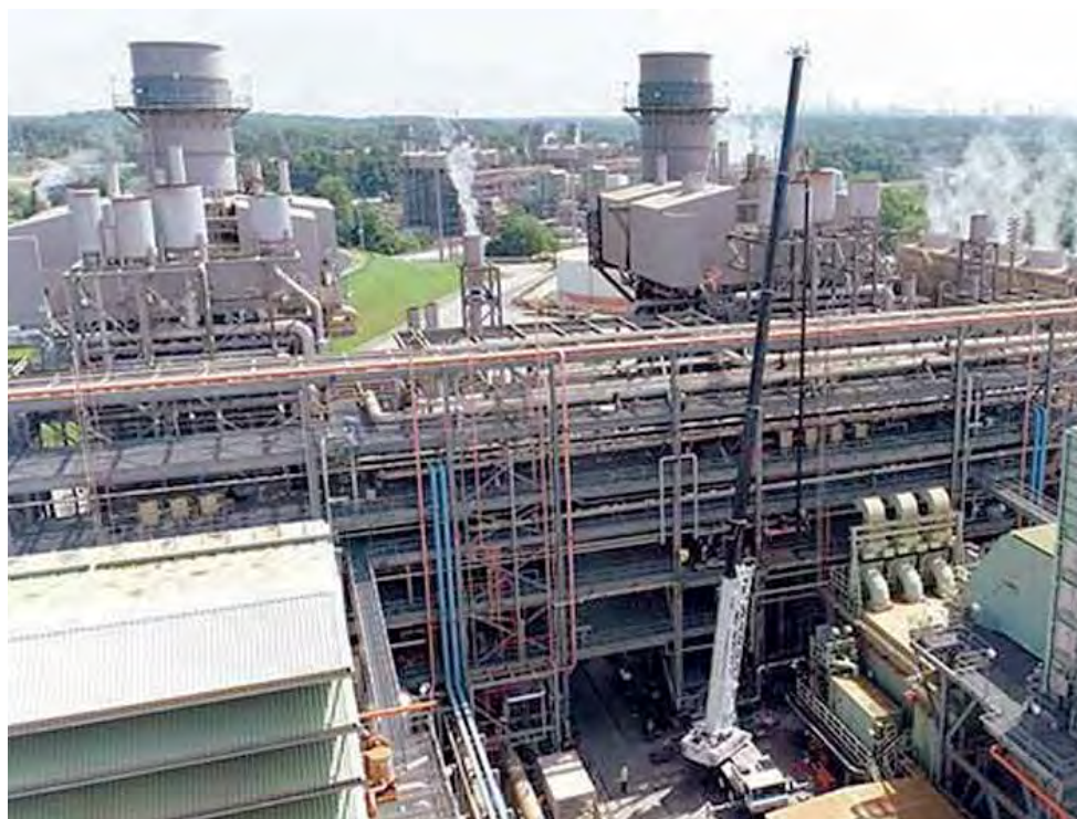
This power plant in Georgia produced electricity with a blend of hydrogen and natural gas during a 2022 test. (Georgia Power)
