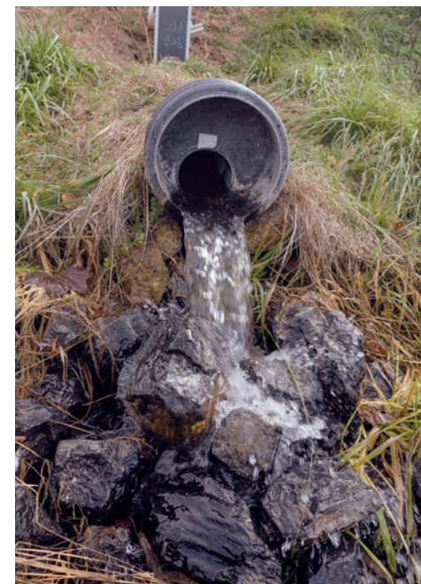
Water from Smith Creek in Rockingham County, VA, flows over a rock pile as it exits a bioreactor and returns to the creek. (Dave Harp)
