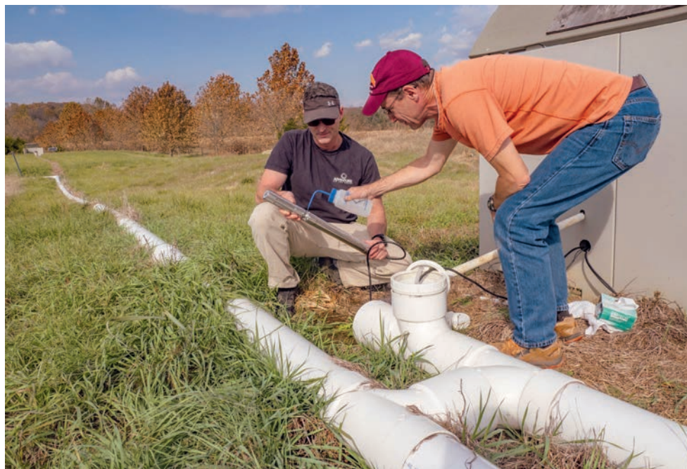
Zach Easton (left) and Kurt Stephenson of Virginia Tech are learning how bioreactors at springs, like the one at the beginning of Smith Creek in Virginia, might help reduce nitrogen loads to the Bay. (Dave Harp)
