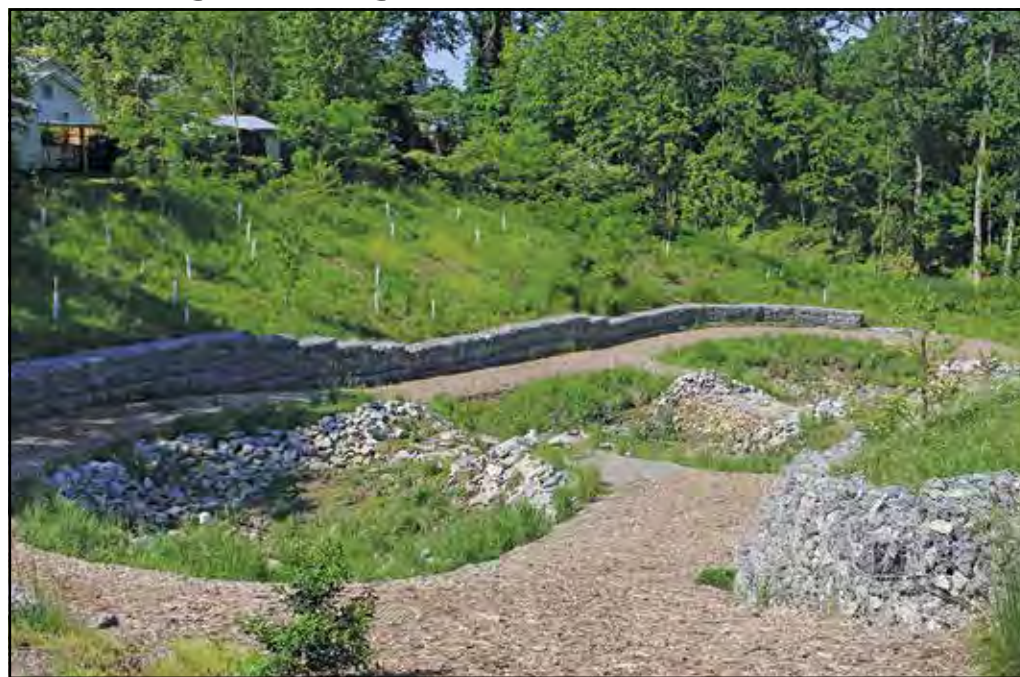
A "regenerative stormwater conveyance system" in Hopewell, VA, controls stormwater runoff from an adjacent neighborhood before it flows into a local stream and out into the Appomattox River. (Sarah Vogel song)
