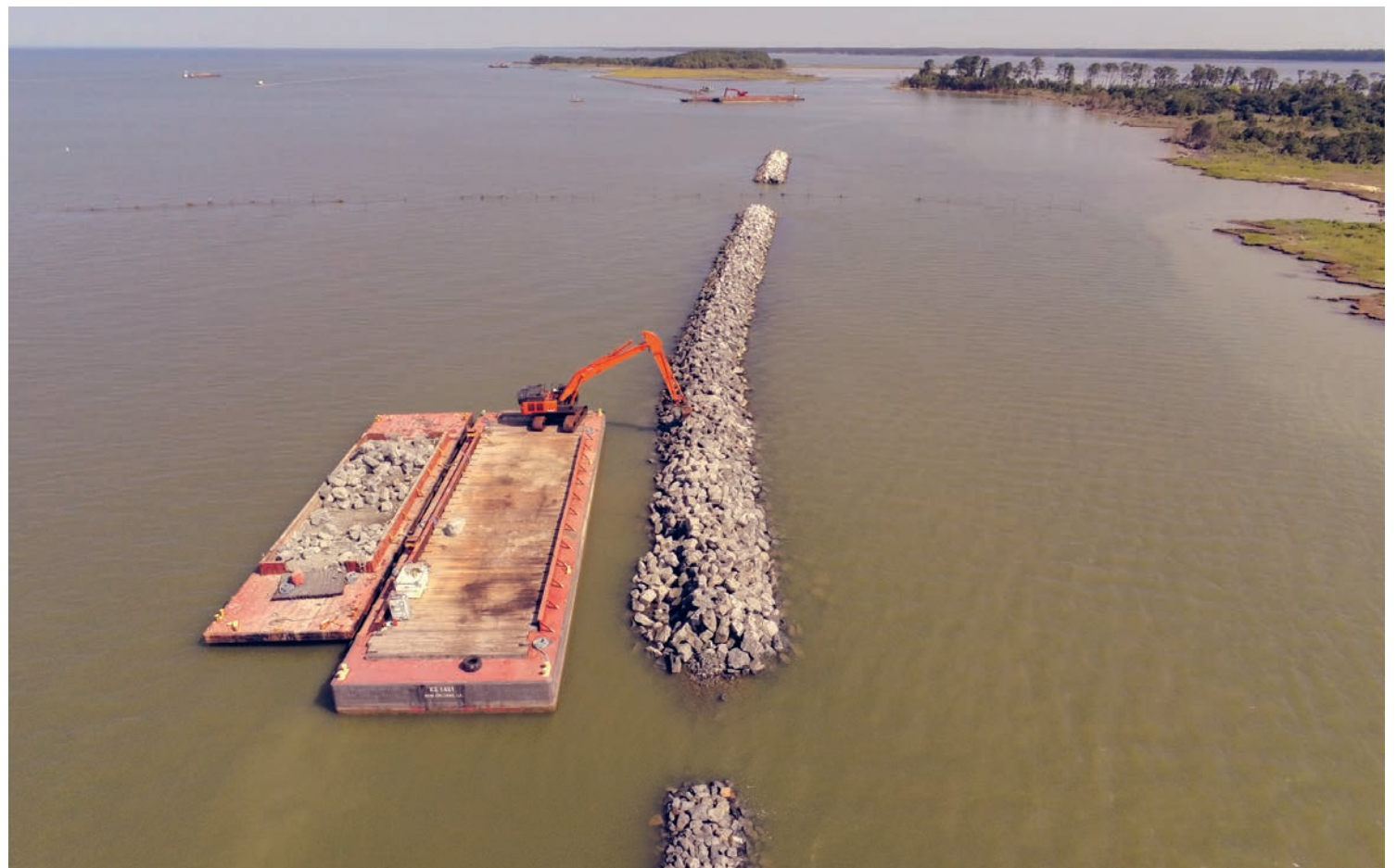
Stone sills rise from the Chesapeake Bay as part of the Barren Island restoration project in Dorchester County, MD. (U.S. Army Corps of Engineers)
